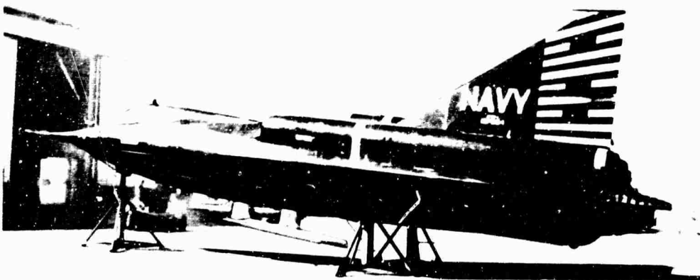
Figure 2-10. Single Small Hydro-Ski Installation on XF2Y-1
