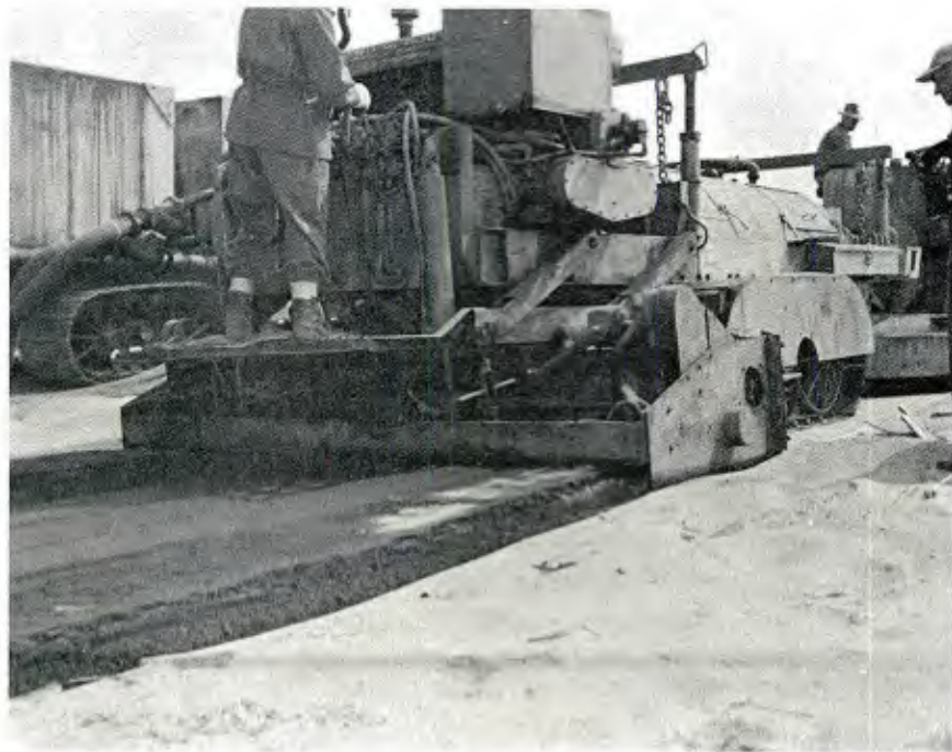
Figure 7. Pressure loading and control of hydraulic vibratory compaction mechanism.
