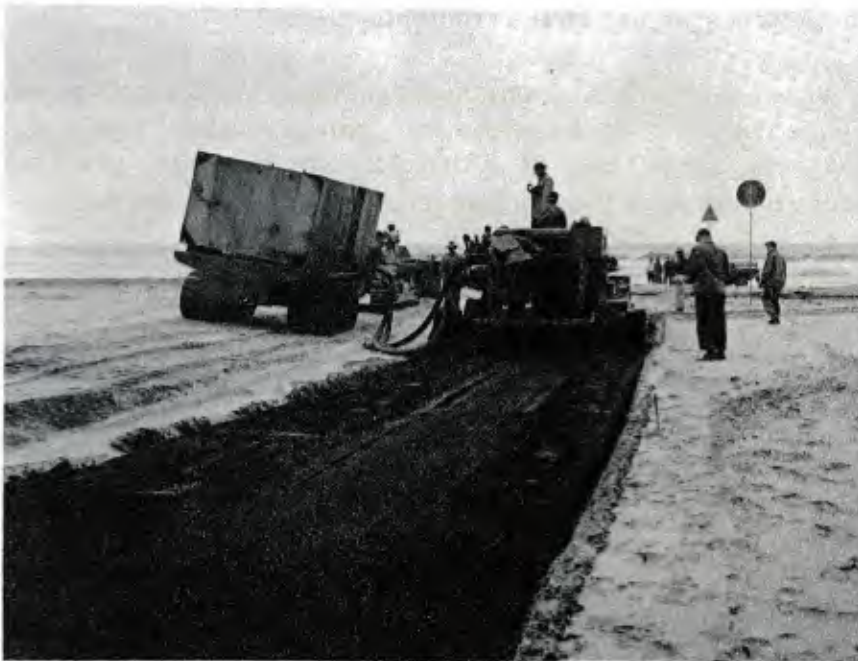
Figure 9. Stabilizing beach sand with chemical mix (note elevation of one side of chemical tank to permit easy draining).
