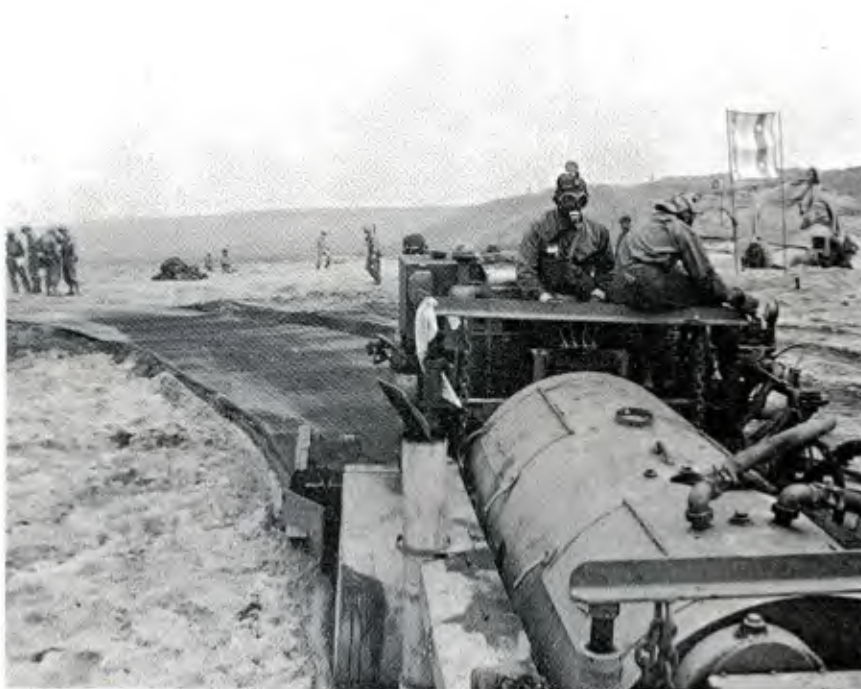
Figure 5. Pug mill with two spray nozzles.
