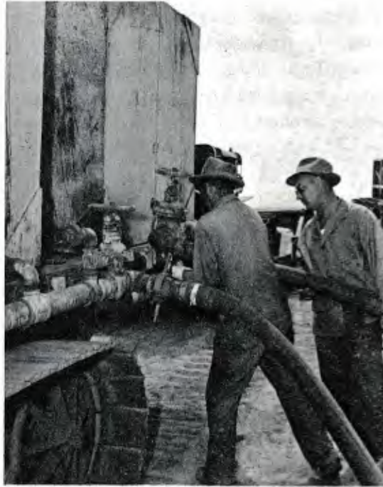
Figure 8. Connecting pump lines to chemical tank.
