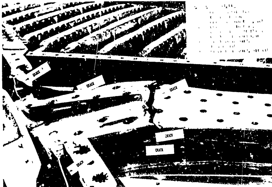
Figure AI.9. Horizontal Stabilizer Test 9; 250°F. Symmetrical; Closeup of Failure of Internal Structure
