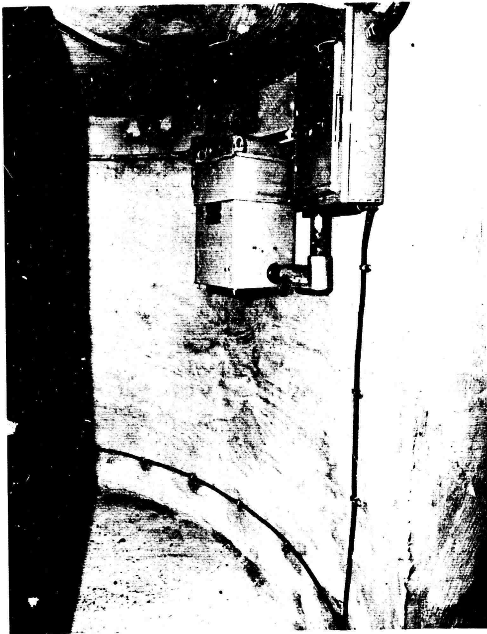
FIGURE 14. COMMERCIAL POWER DISTRIBUTION UNITS, CTH
