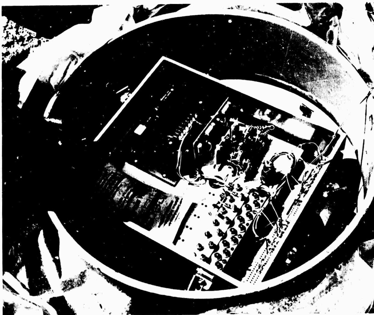
FIGURE 18. WELL HEAD VAULT, HOFFMAN BOX, COVER REMOVED
