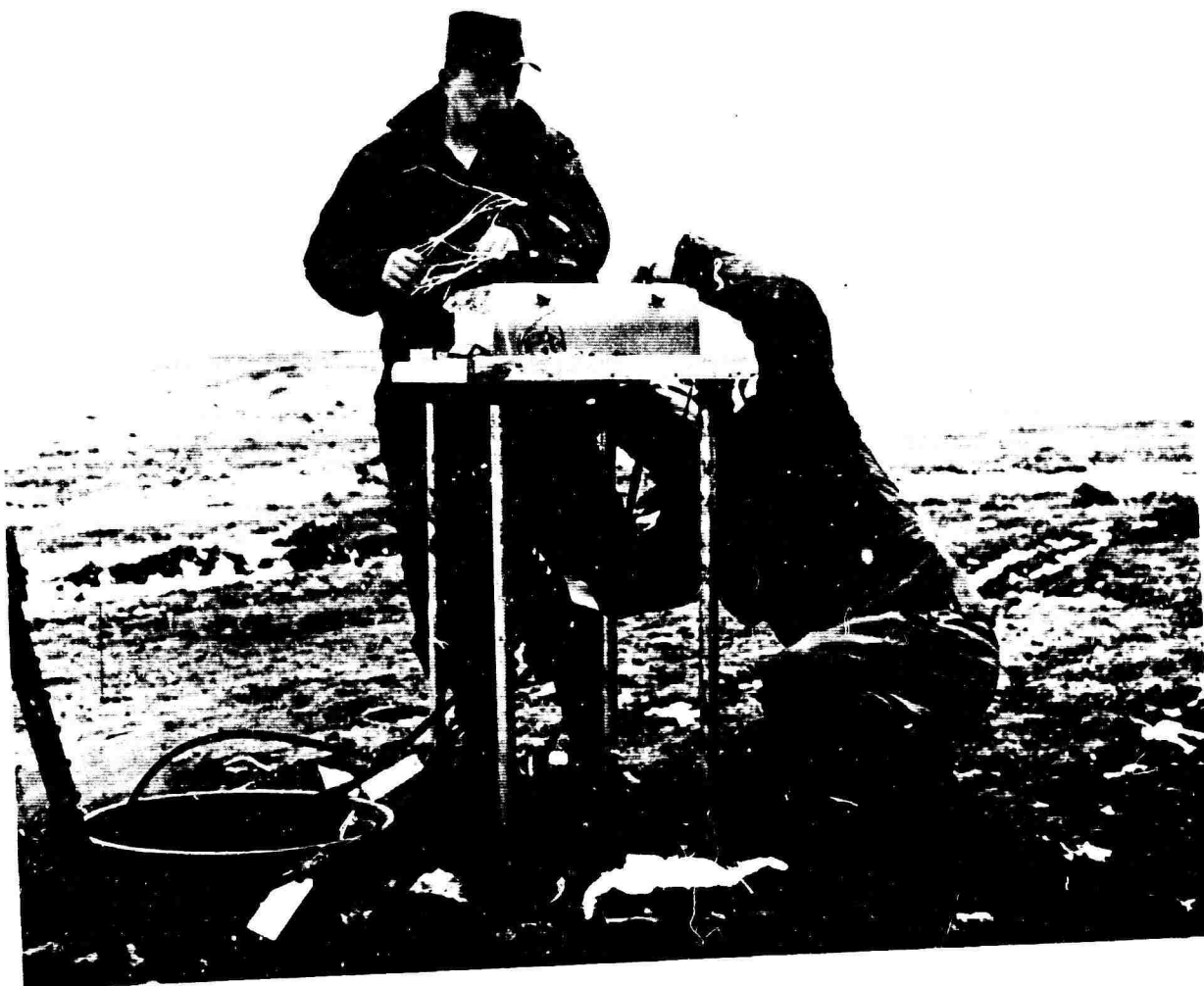
FIGURE 29. INSERTING CABLES INTO JUNCTION BOX
