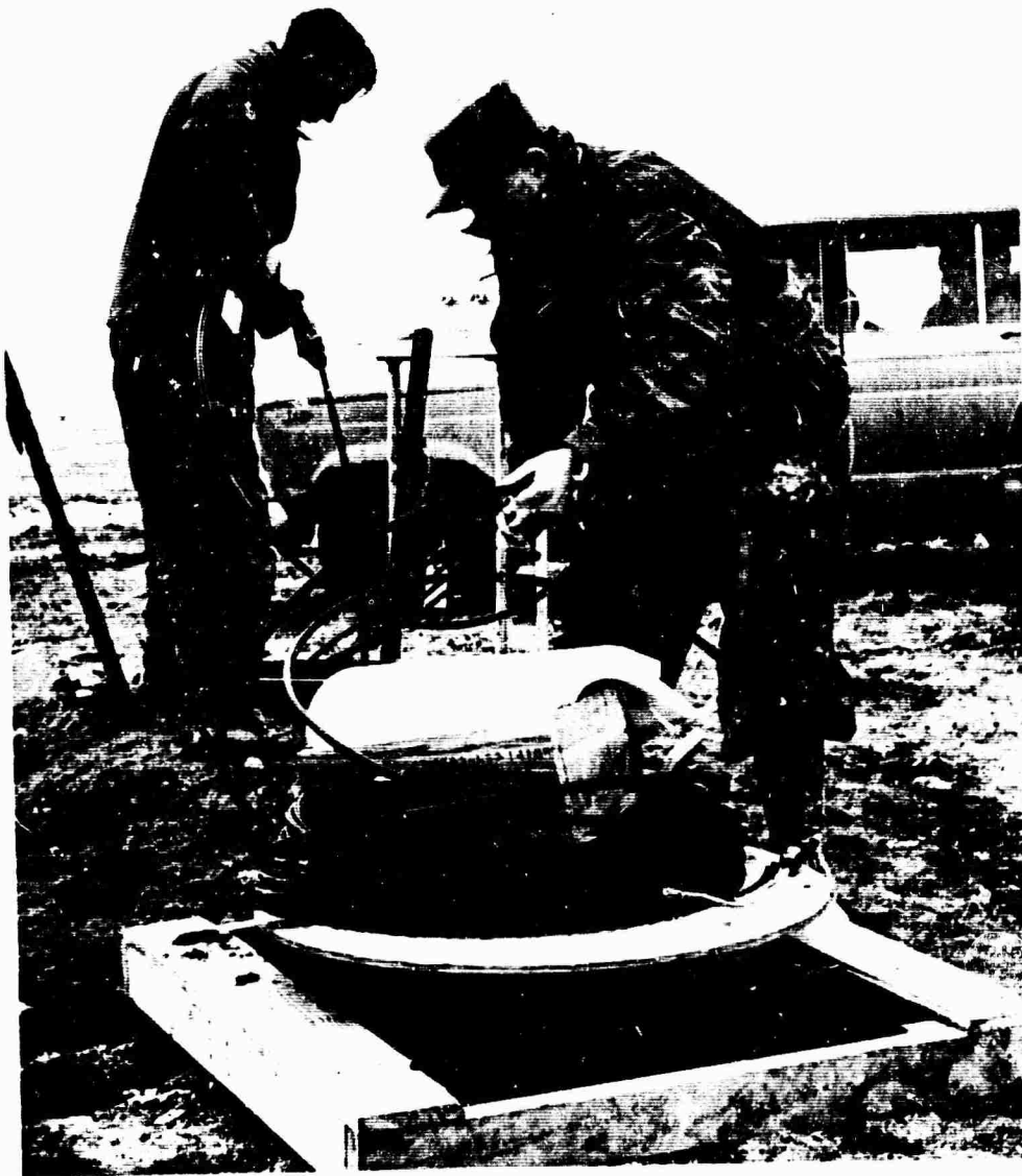
FIGURE 28. EMPLACING SEISMOMETER IN CASED HOLE
