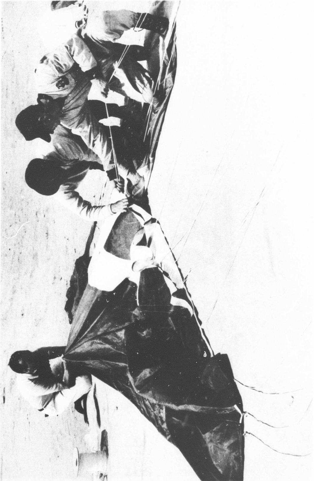
Figure 4. Pleating and Line Stowage of Parawing (Start).
