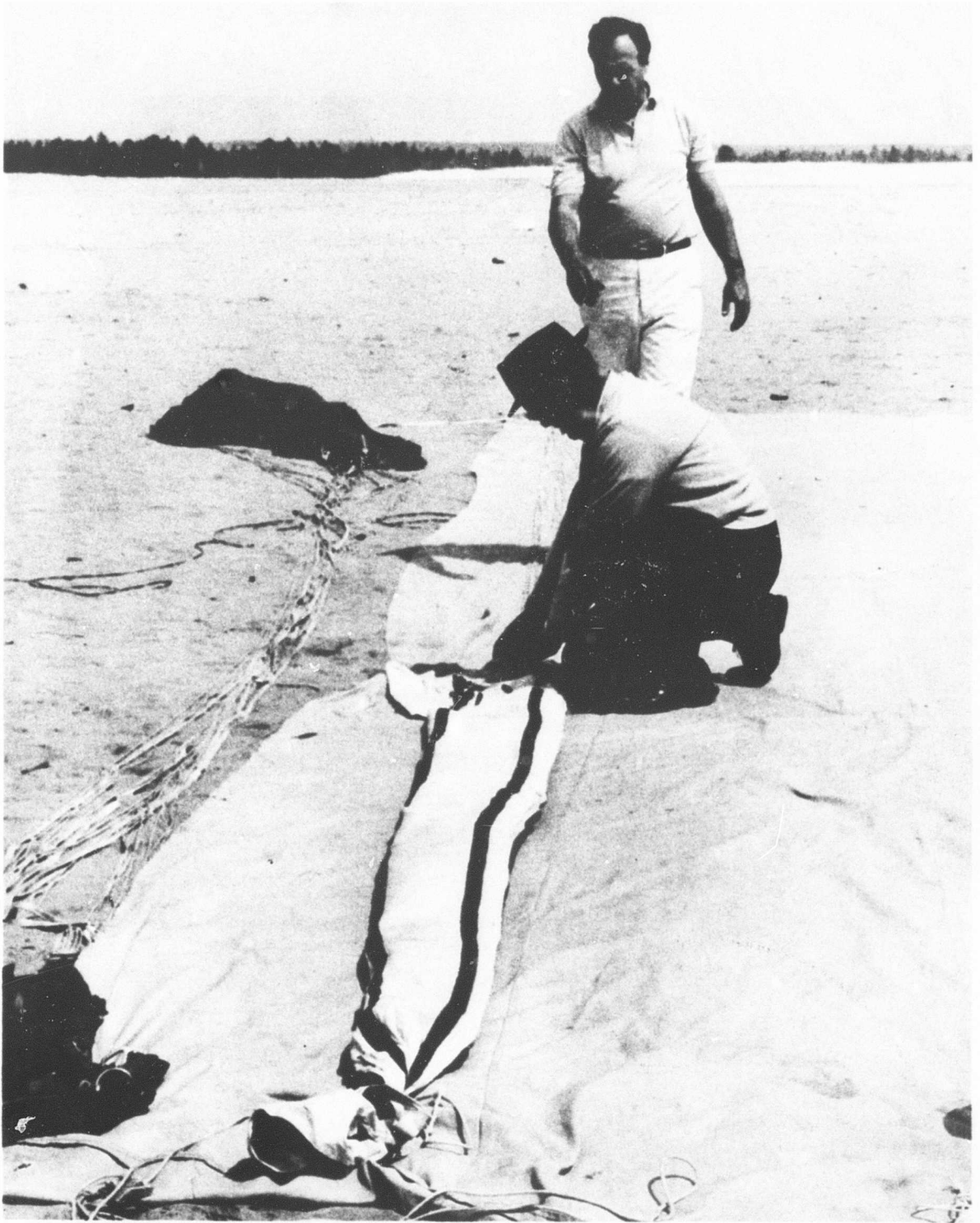
Figure 9. Parawing Stowed in Sleeve.
