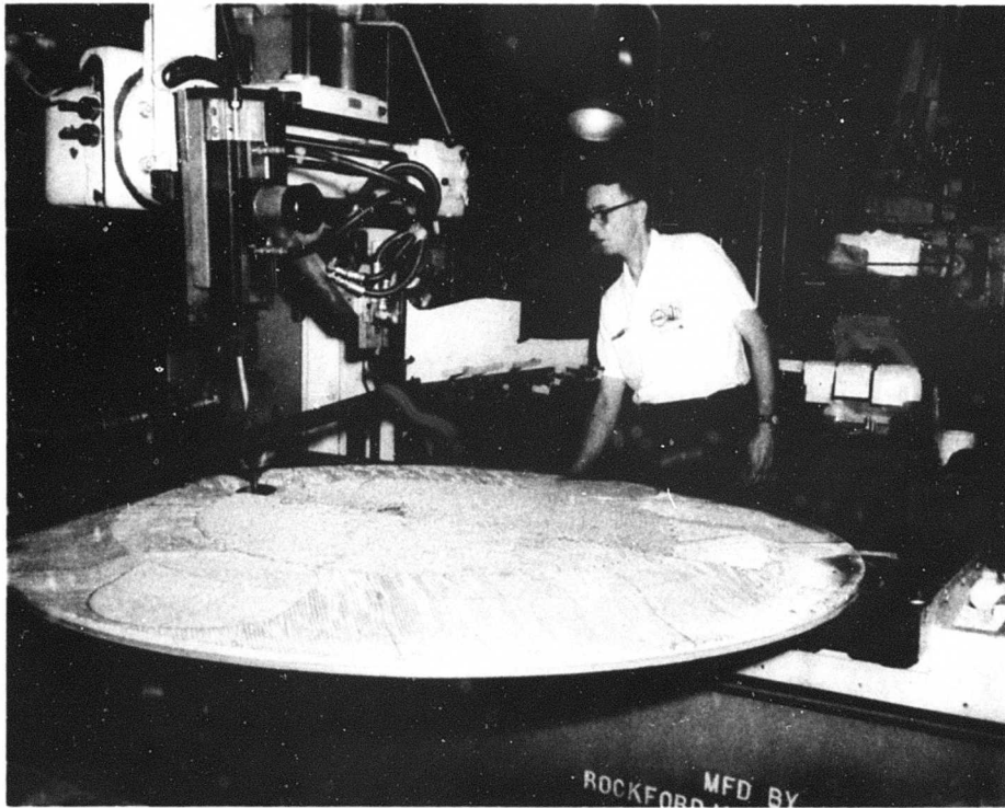
Figure 4 Honeycomb Core - Wing Fan Door
