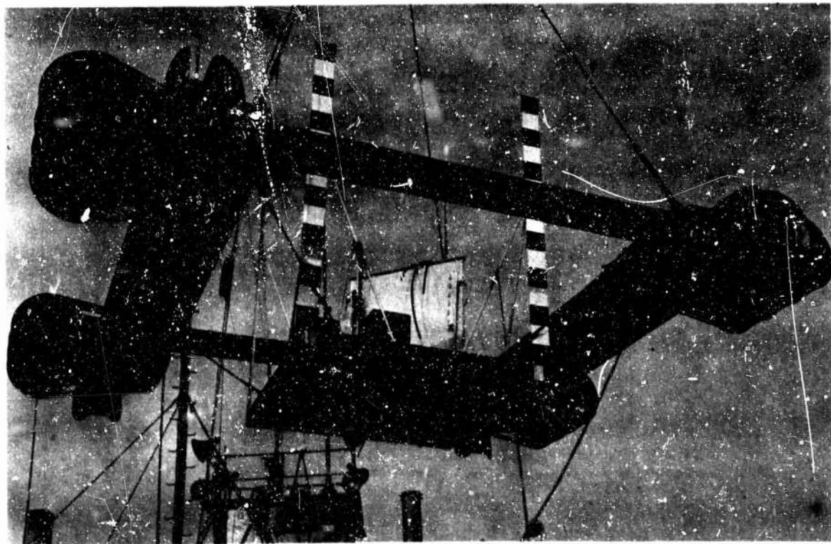
Figure 2 - Light Wooden Float Within Work Platform
