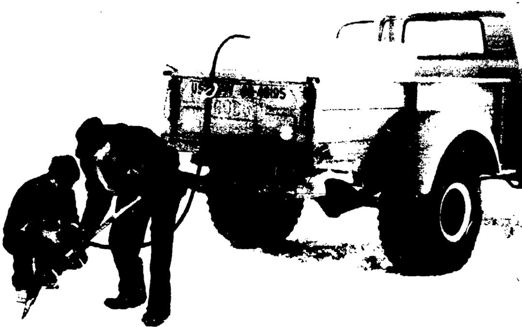
Figure 8. Making a water patch during DF-65 trials.
