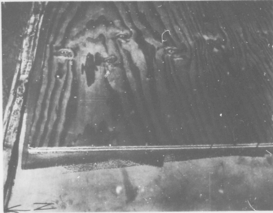
Figure 6. Plywood cemented to sheet-metal sections used in construction of ceiling. Elevator bolts shown do not penetrate sheet metal.
