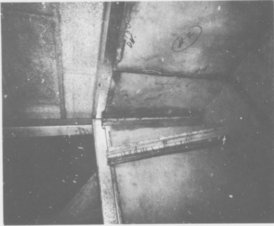
Figure 9. Southeast corner of shielded building showing detail of sheet-metal strip used at the corner seams. Also shown is a strip not yet in place.
