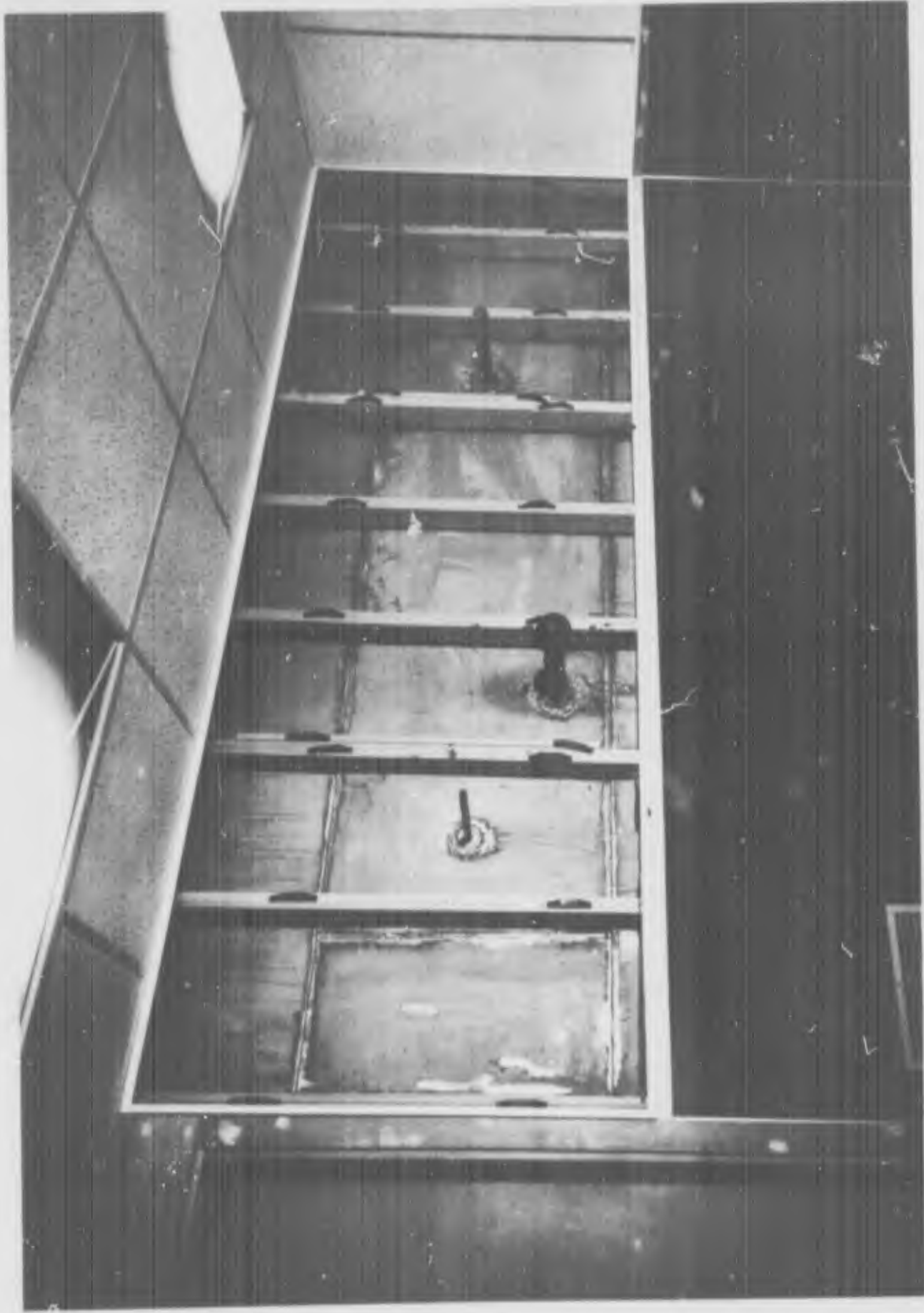
Figure 22. North wall of shielded room showing the acoustic tile removed and the three pipe penetrations mounted in positions suitable for tests.
