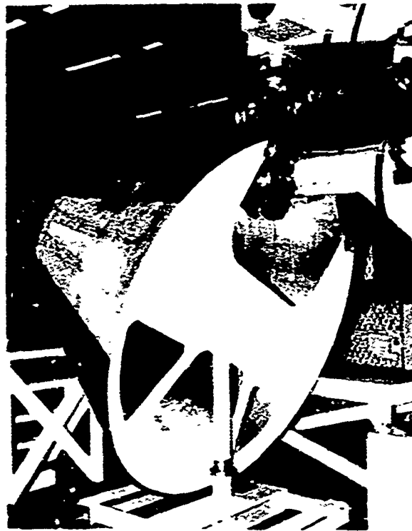
FIGURE 87. INNER AND OUTER MERCURY CAPSULE SKINS ARE SEAM WELDED (REF. 91)
