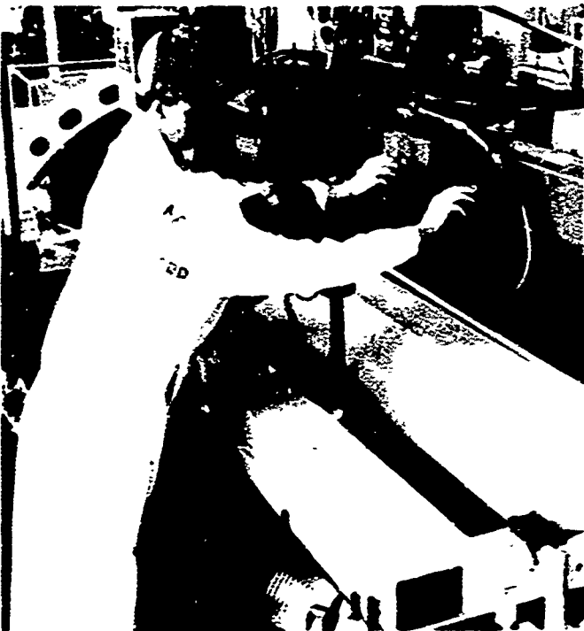
FIGURE 42. FIXTURE HOLDS FIRST TWO PANELS OF OUTER CONICAL SKIN FOR TIG WELDING (REF. 52)
