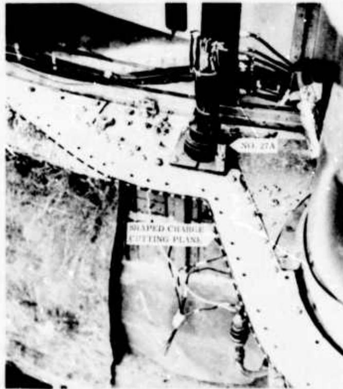
Fig. 6. Accelerometer on electrical wiring staging disconnect
