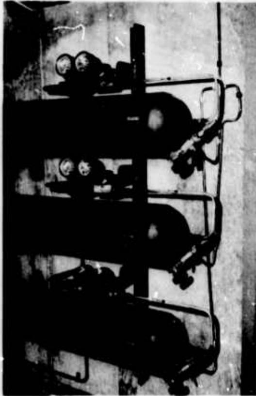
Fig. 5. Compressor room regulators and receivers
