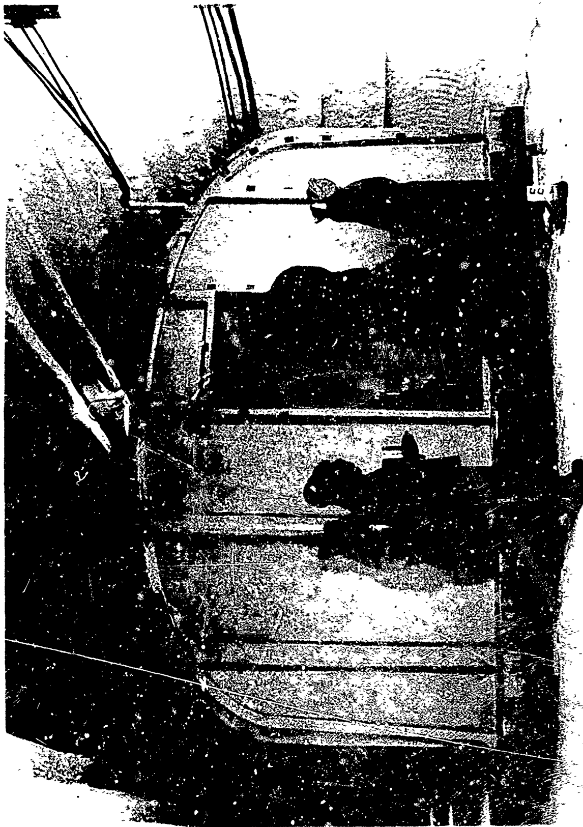
Figure 1. Glass Fiber, Polyurethane Plastics Building Located in a Snow Tunnel.
