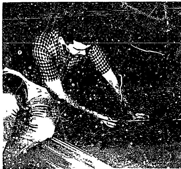
FIGURE 47: Frame being rotated into triangular "keystone" section.
