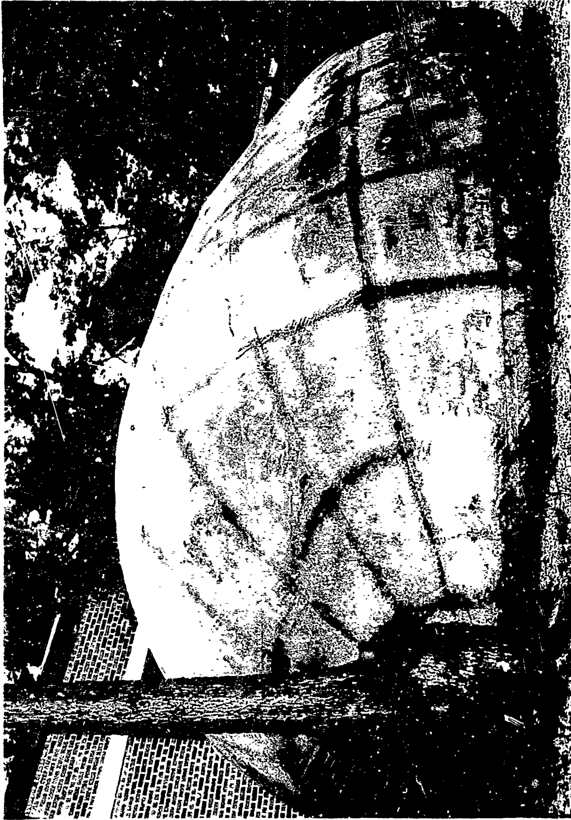
Figure 14. Exterior of Sprayed Shelter. The Structure Consists of A 3" Foam Core with Interior and Exterior Skin of Reinforced Plastic
