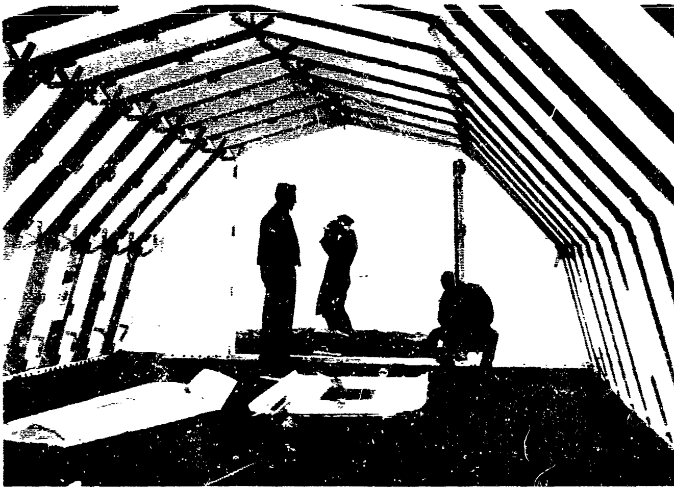
FIGURE 37. SHELTER #2 FIELD TEST, LANGLEY AFB (INTERIOR VIEW SHOWING INSTALLATION OF END COMPONENTS)
