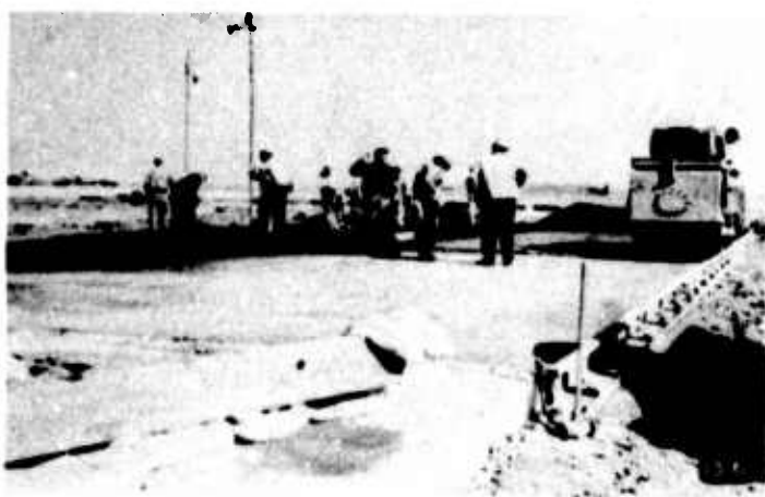
(b) ROLLING SAND-ASPHALT CUSHION IN SECTIONS M & L. 10-20-43.
