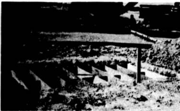
(b) TYPICAL GANG FORM AT SECTION Y 1 FOR FIELD CURED CONTROL BEAMS. 9-29-43.
