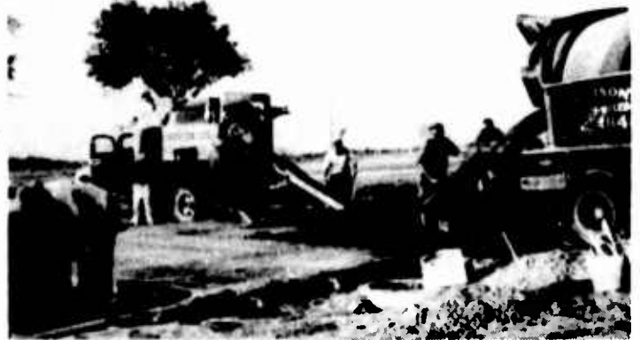
(a) MIXER TRUCKS PLACING CONCRETE IN LANE 1 OF WEST TURN AT SECTION U. 8-30-43.
