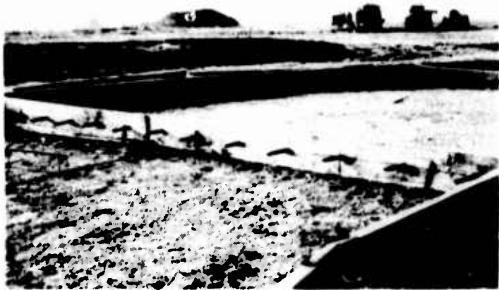
(a) TIMBER BULKHEAD FOR TRANSVERSE DOWELED CONSTRUCTION JOINT LANE 1, BETWEEN SECTIONS V 1 & V 2 , EAST TURN. 10-1-43.
