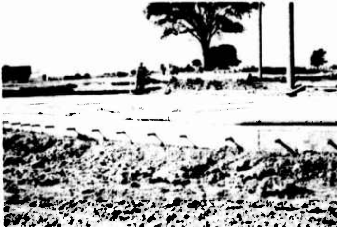
(b) LONGITUDINAL DOWELED CONSTRUCT- ION JOINT BETWEEN LANES 1 & 2, SECTION W 2 , EAST TURN. 10-7-43.
