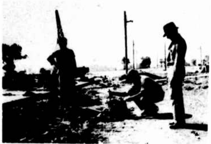
(a) (1) SLUMP TEST. (2) BEAM GANG MOULDS FOR FIELD CURING. (3) DOUBLE BEAM MOULD FOR LAB. CURING. 10-1-43.
