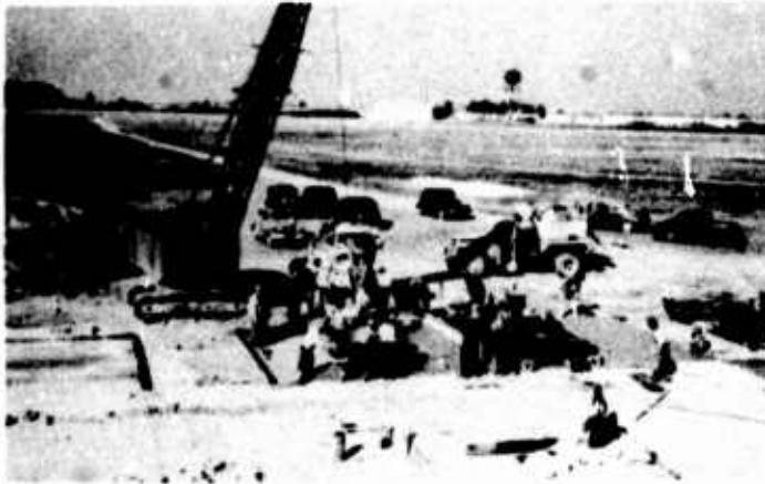
(b) GENERAL VIEW OF CONCRETING OPERATIONS, STATIC SECTION F, SHOWING CRANE, EQUIPPED WITH BOTTOM DUMP BUCKET, PLACING CONCRETE. 10-19-43.
