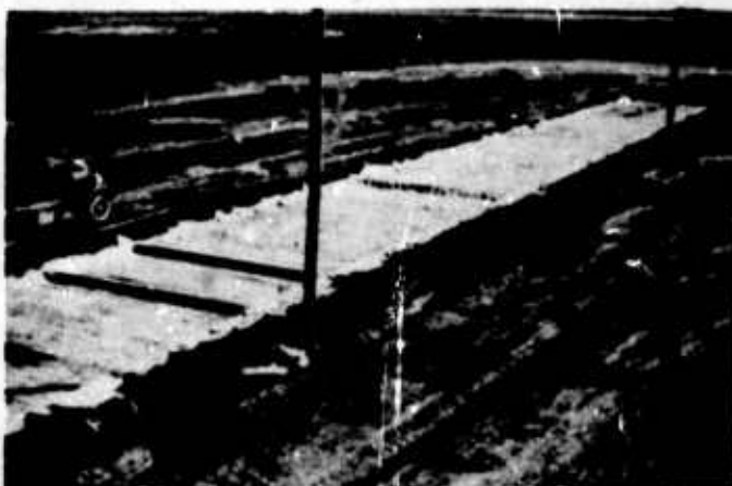
(c) VIEW ALONG NORTH SIDE OF TRACK, LOOKING EAST FROM CUPOLA, SHOW- ING COTTON MATS PROTECTING FINAL GRADE PRIOR TO CONCRETING. 9-29-43.
