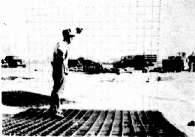
(c) 65# WIRE MESH REINFORCING 6"X6" MESH IN SECTIONS 9-8'X10'-6". 10-21-43.
