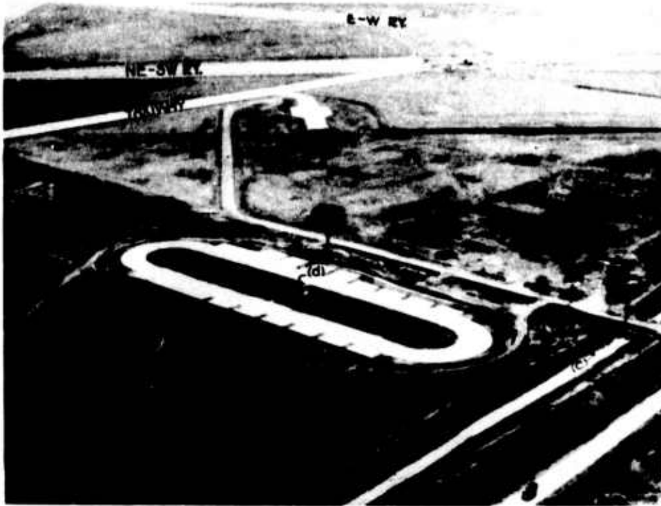
DISTANT VIEW SHOWING: (a) TRACK SHORTLY AFTER COMPLETION. (b) LOCATION WITH RESPECT TO FLYING FIELD. (c) CONNECTION TO DRAINAGE DITCH. (d) FIELD OFFICE.
