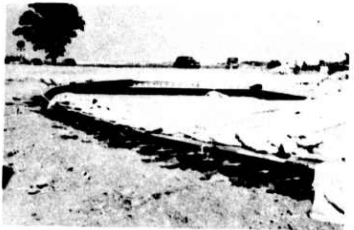
(c) LONGITUDINAL CONSTRUCTION JOINT WITH TIE BARS, PRIOR TO STRIPPING FORMS, BETWEEN LANES 1 AND 2, SECTION W 2 , WEST TURN. 9-30-43.
