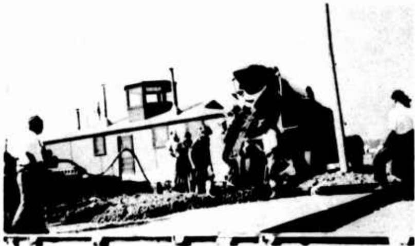
(a) CONCRETE PLACEMENT IN LANE 1, SECTION Q. 10-1-43.
