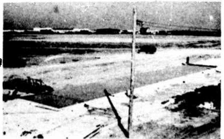
(c) VIEW OF COMPLETED SECTIONS G, H, J, LANE 2, SHOWING FINISHED PAVE- MENT BEING COVERED WITH COTTON MATS FOR CURING. 10-19-43.
