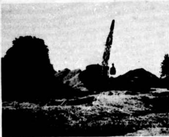
(a) STOCK PILES OF SELECTED SUBGRADE AND BASE COURSE MATERIALS. MATERIALS, FROM LEFT TO RIGHT, SELECTED SUBGRADE, PLUME SAND & BANK-RUN SAND & GRAVEL. 9-7-43
