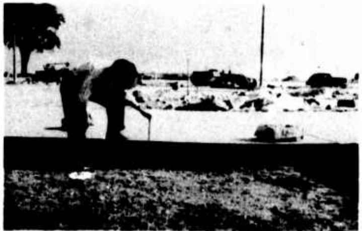
(c) KEYED LONGITUDINAL CONSTRUCTION JOINT BETWEEN LANES 1 AND 2, WEST TURN, SECTION Y. 10-7-43.
