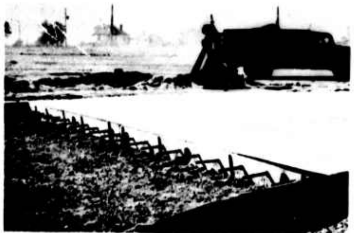
(a) TRANSVERSE CONSTRUCTION JOINT WITH TIE BARS, BETWEEN SECTIONS 2, AND 2 2 , LANE 1, WEST TURN. BULKHEAD IN PLACE. 9-30-43.
