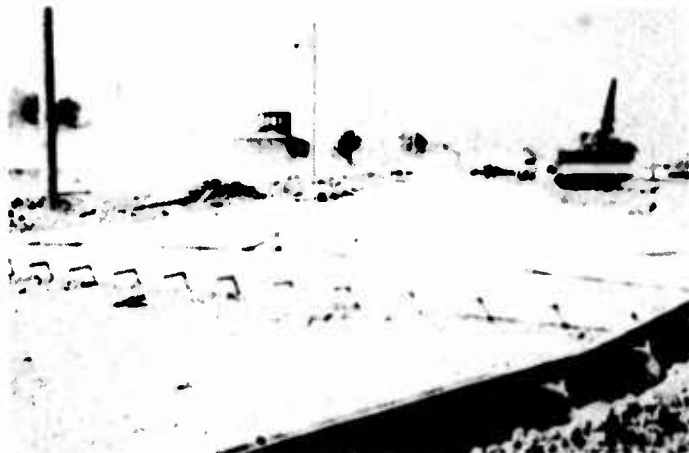
(c) TRANSVERSE DOWELED CONSTRUCT- ION JOINT BETWEEN SECTIONS X 1 AND X 2 , LANE 1, EAST TURN. 10-7-43.
