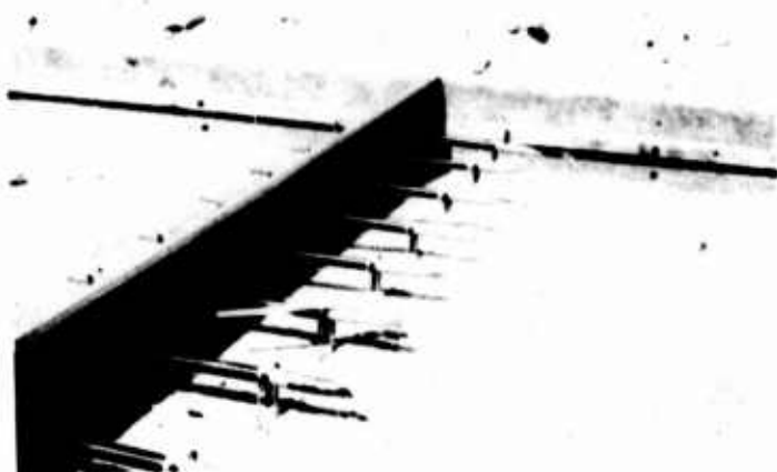
(b) VIEW SHOWING DETAILS OF TRANSVERSE DOWELED EXPANSION JOINT IN PHOTOGRAPH (a). 9-29-43.
