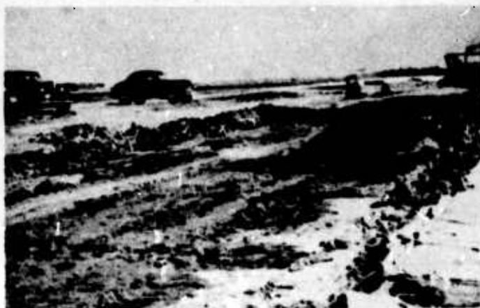
(b) ROUGH EXCAVATION OF LANE 2, SECTION B, SHOWING SOFT SPOT IN SUBGRADE. 10-1-43.
