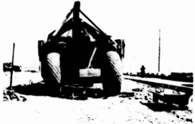
(a) FIELD BEARING TEST SETUP USING 10 YD CARRIMOR SCRAPER FOR LOAD REACTION. 10-21-43.
