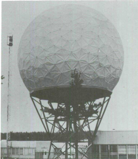
The space-frame radome of the Bedford interferometer site houses the steerable radar antenna which both transmits and receives for two-site interferometry. For three-site interferometry the antenna receives radar returns from the Millstone Hill radar transmitter. In the background is the antenna tower for the microwave link which is used for synchronization of the three radar sites and for centralized collection of the radar returns.
