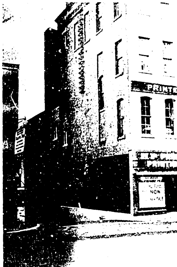
View of Building from Intersection of South Avenue and Ely Street
