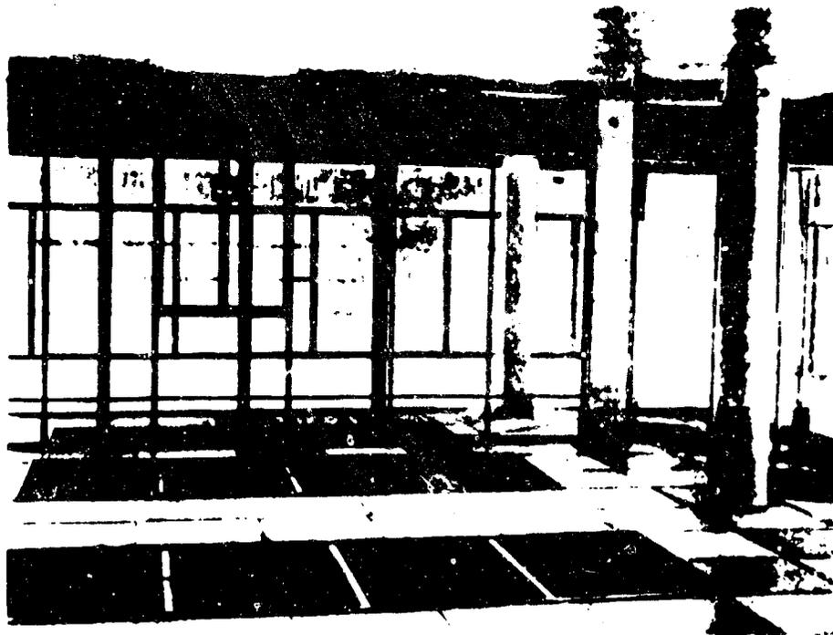
Fig. 10. Aluminum partitions and suspension ceiling of experimental building.
