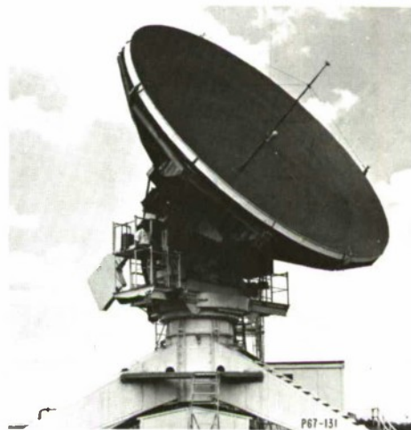
Fig. 16. The 28-foot precision parabola developed using spin-casting techniques.
