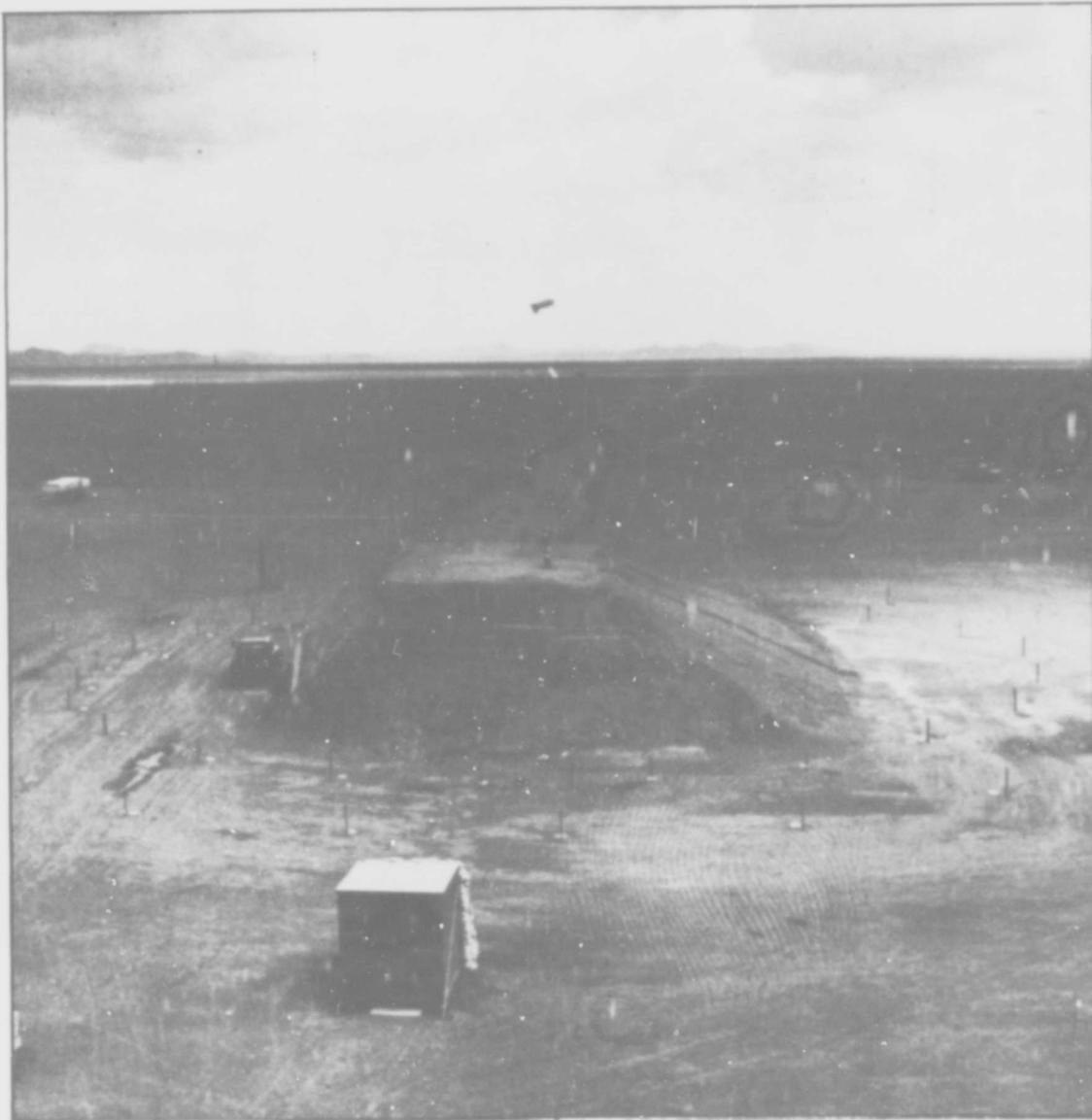
FIG. 85. Igloos Covered With Eight Feet of Earth, Roller Coaster Test.
