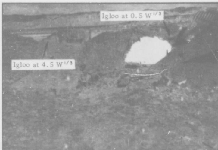
FIG. 7. Magazine After Firing Test.
