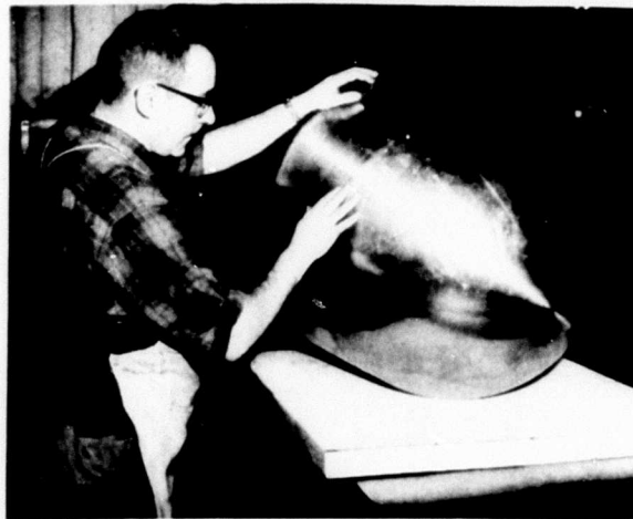
Figure 1. RE-ENTRY VEHICLE Hemisphere - Mo-TZM; Frustum and Fairing - Inconel X
