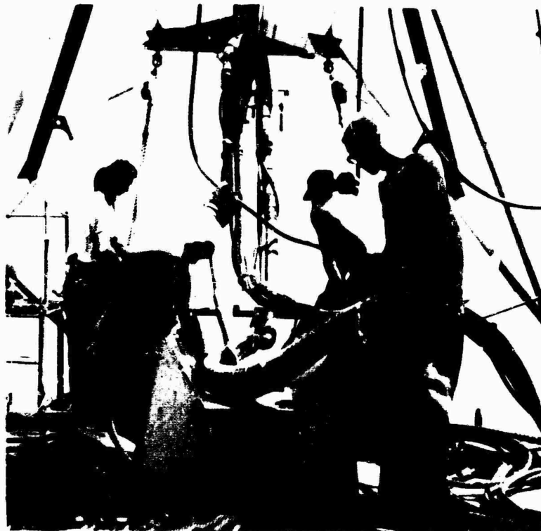
Fig. 13 - Umbilical cord being lowered to Sealab
