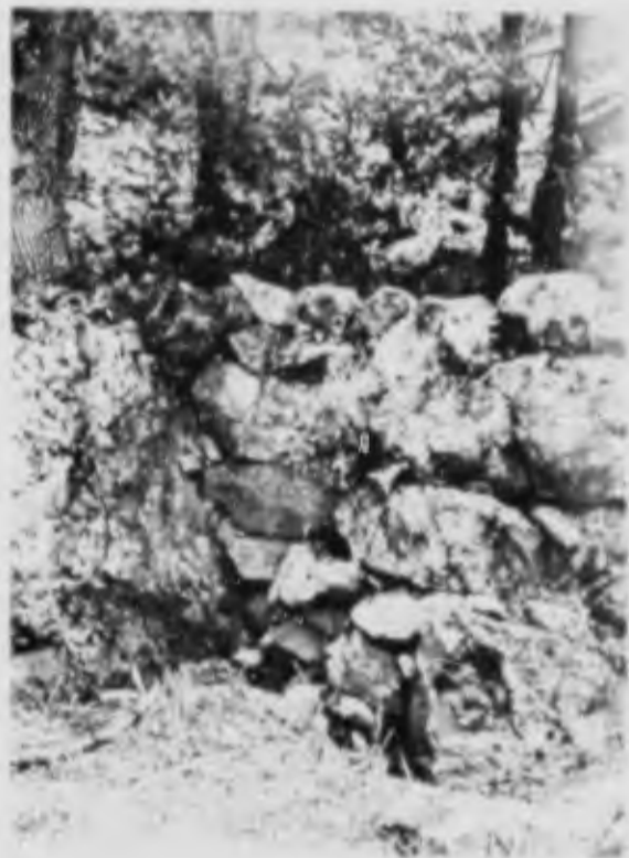
Photograph 14. Abutment of Check Dam 434 with Bedrock Outcrop. Height 4 Feet.
