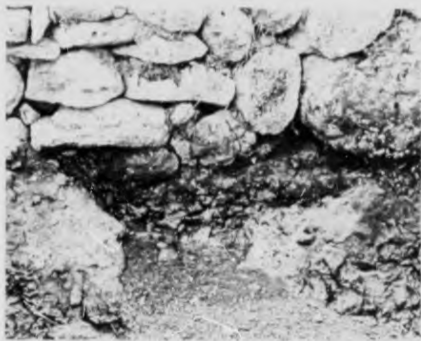
Photograph 15. Contact of Base of Trinchera Wall 319 with Bedrock. A Small Pool of Water has Collected Here.
