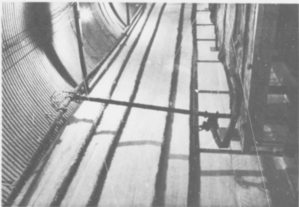
Figure 34. Typical result of placing a rigid member between the trench floor and the roof. As the wall deforms, the vertical pipe distorts the horizontal pipe to which it is connected, and itself begins to buckle. (Official U. S. Navy photograph)
