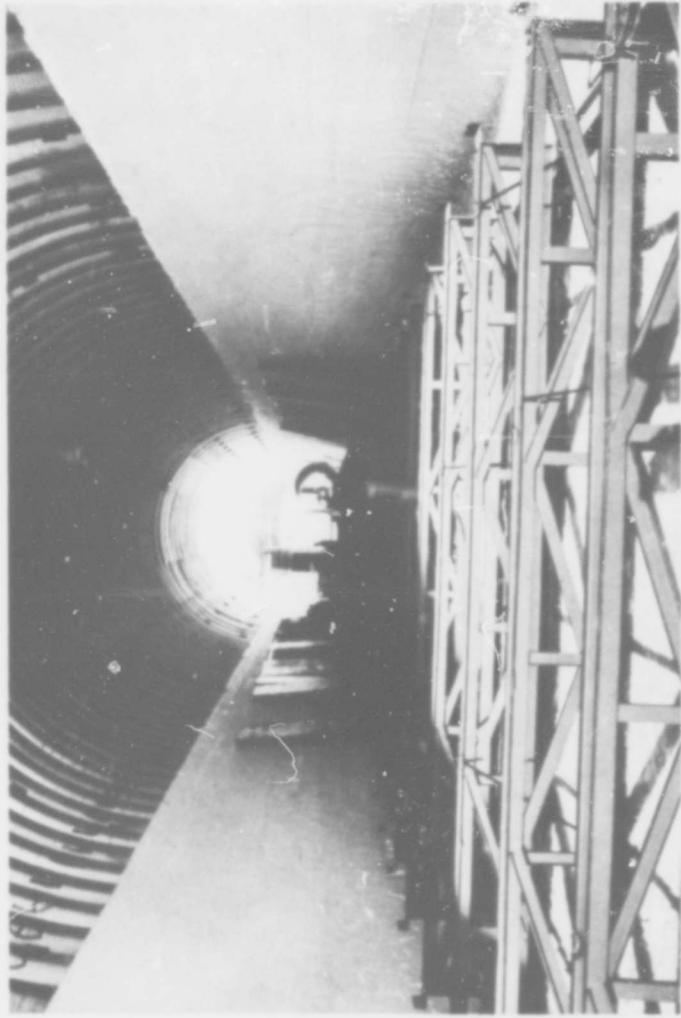
Figure 3. Foundations for the meteorology building in trench L-8. The open-web joists span between timber sills. (Official U. S. Navy photograph)
