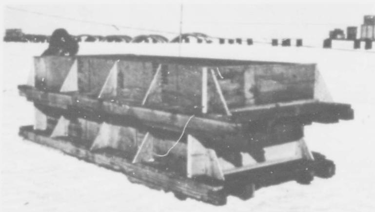
Figure A1. Casting beds for processed snow beams.
