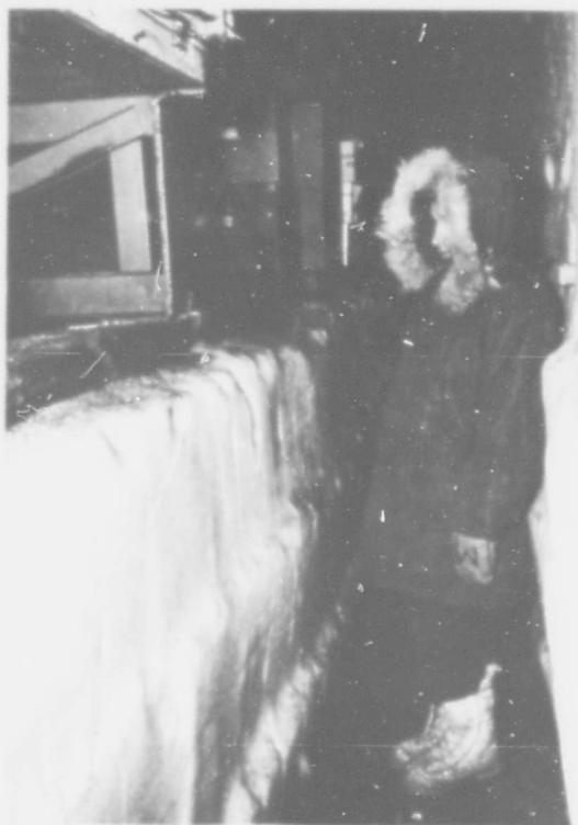
Figure 36. Sewer trench cut alongside the foundation of the meteorology building in trench L-8. Excavating so close to a foundation is bad practice. (Official Navy photograph)
