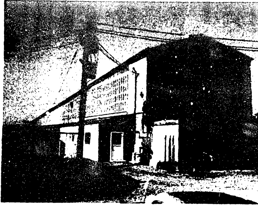
Fig.1 Exterior view of fog chamber. The building is 820 ft. long by 30 feet wide. The height varies from 30 ft. high in the foreground to 10 ft. at the midpoint.
