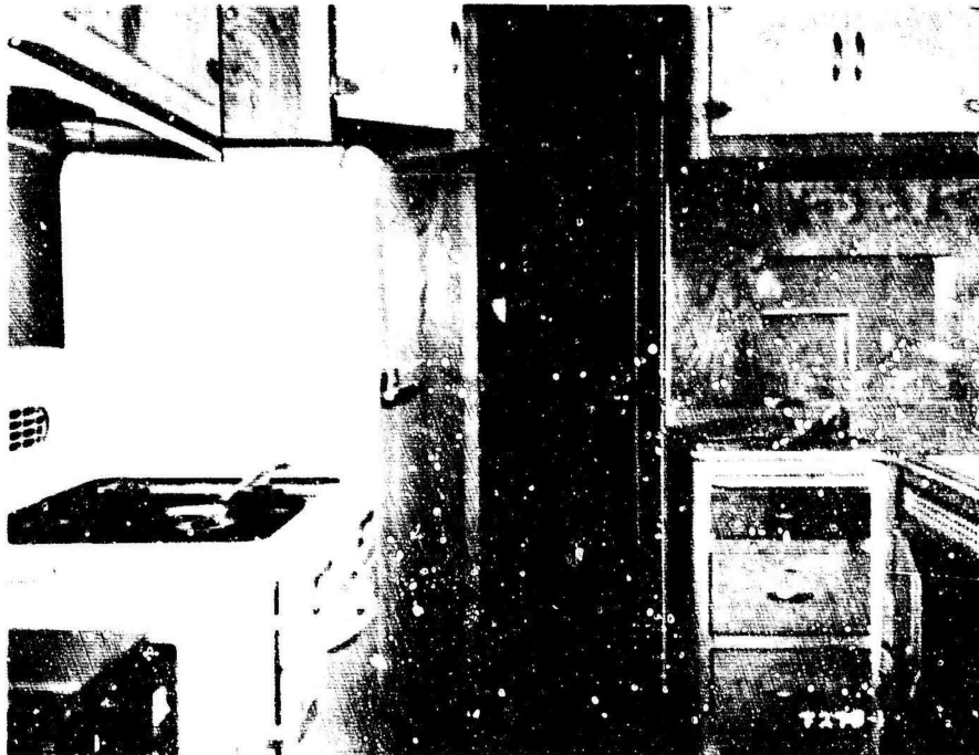
Fig. 2.14—interior of Columbia trailer after the blast.
