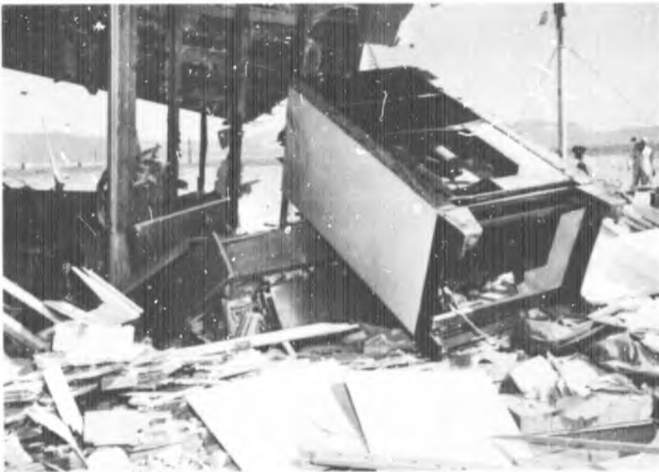
Fig. 29—Wreckage of kitchen showing food shelves in brick house at 4700 ft after the explosion.
