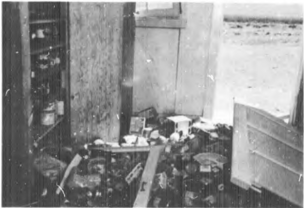
Fig. 33—Wreckage in kitchen of frame house at 5500 ft. Many foods were thrown to floor causing some breakage.
