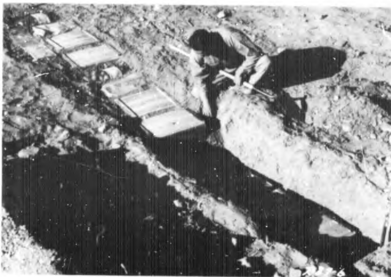
Fig. 2—Trench at Station A (1100 ft) showing arrangement of semiperishables at different depths before covering with soil, Shot L.
