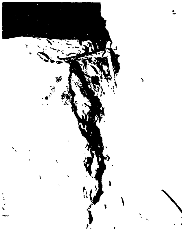
Fig. 3.21 — Detail view of chipped-out section at top of entrance facing away from GZ.
