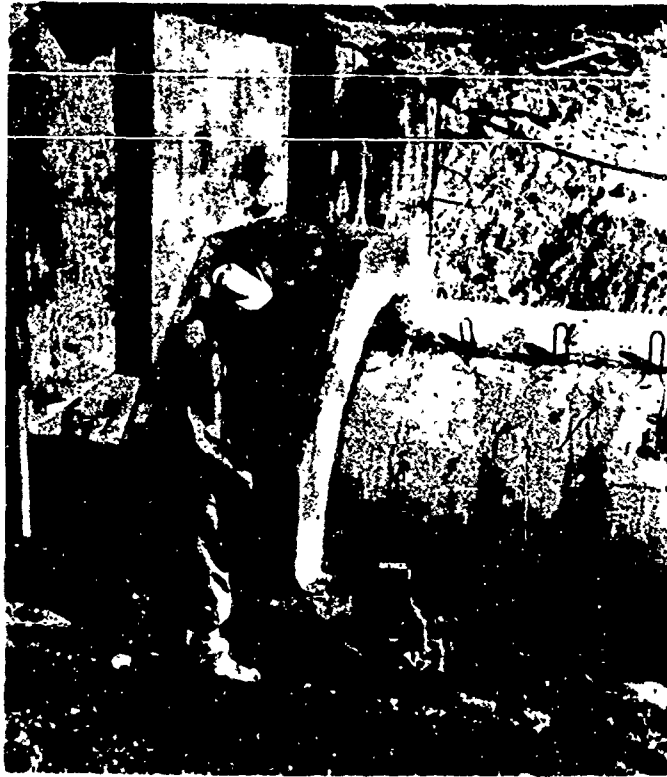
Fig. A.11—Structure II-2, standard compaction procedure near structure (Aug. 7, 1957).
