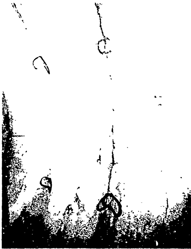
Fig. 3.27 — Spalling and cracking on GZ side of ring 10.
