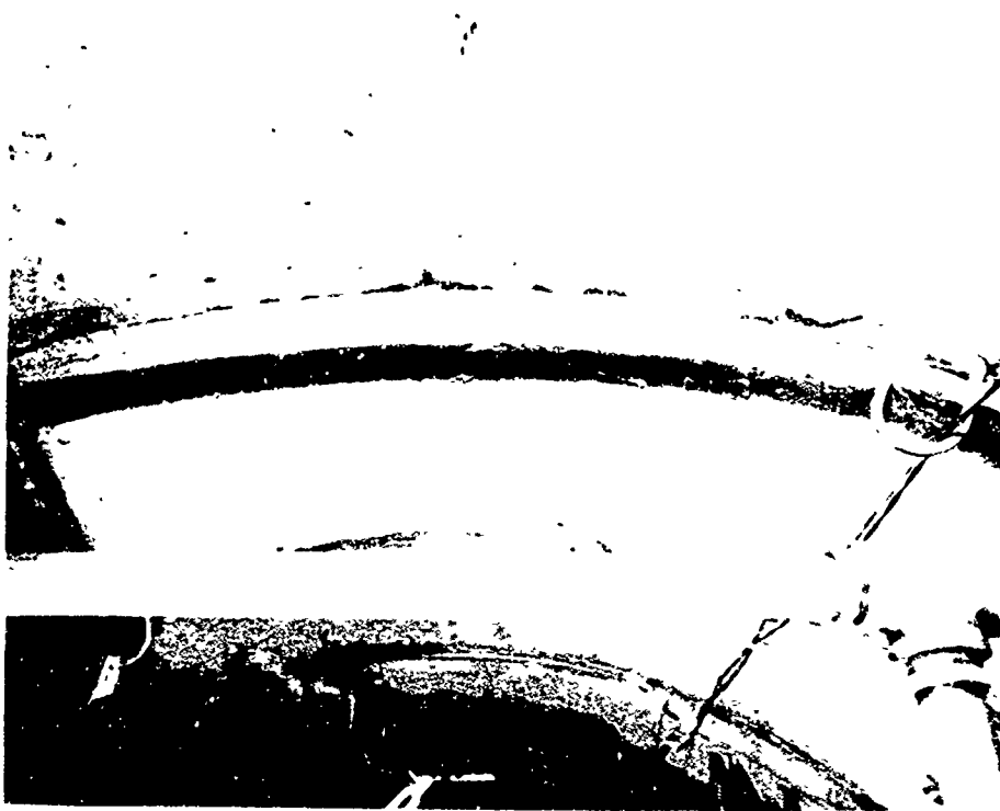
Fig. 3.29 — Vertical movement of ring 10 in relation to ring 11 at their crowns.
