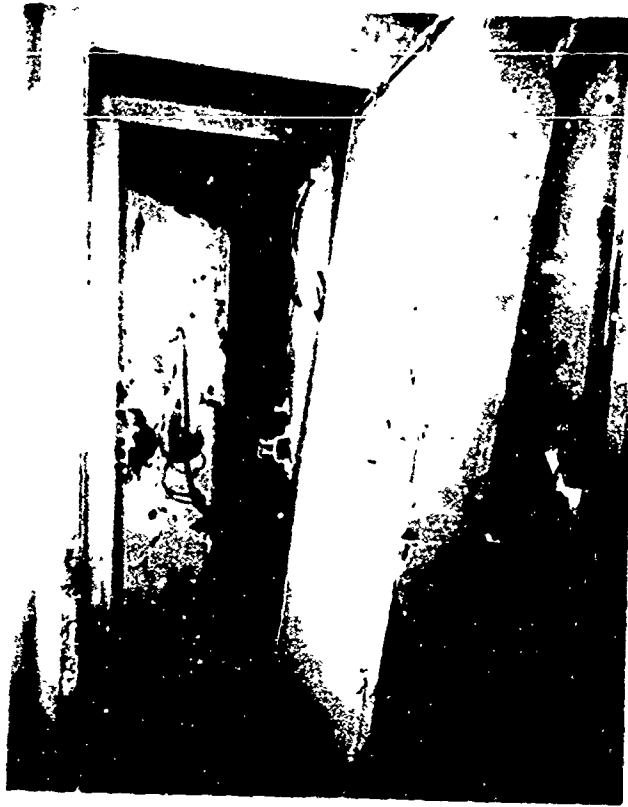
Fig. 3.14 — Blast damage of main entrance.
