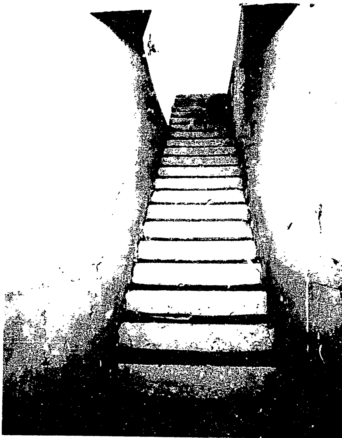
Fig. 3.56— Blast debris deposited on stairs of entrance facing away from GZ.
