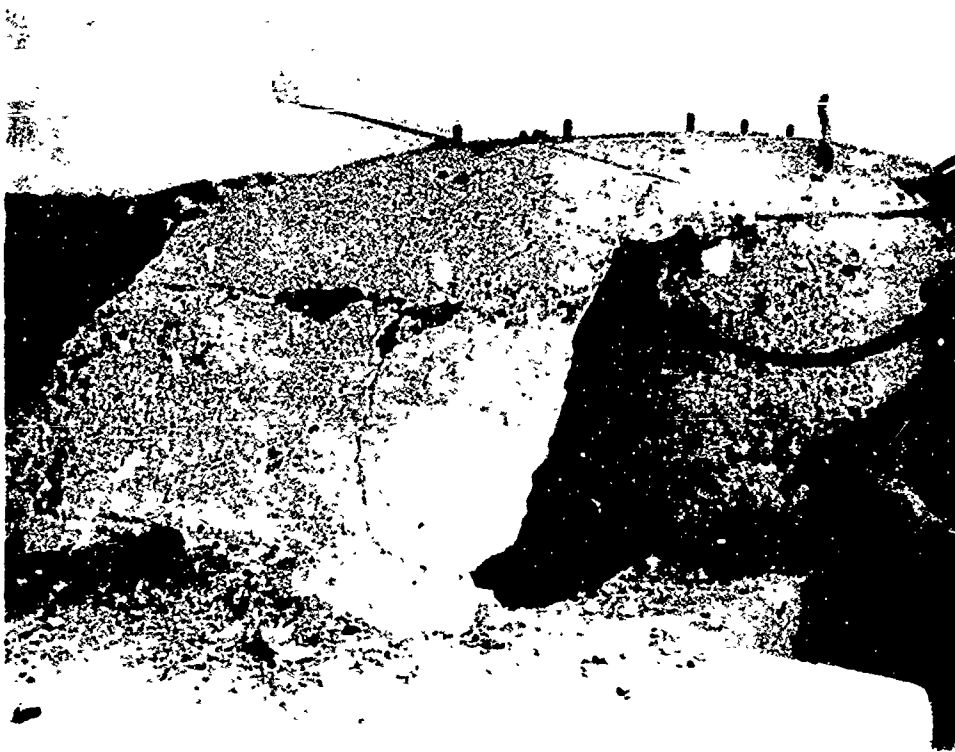
Fig. 3.41 — Blast damage to exposed surface of front reflection shield of sand-pit.
