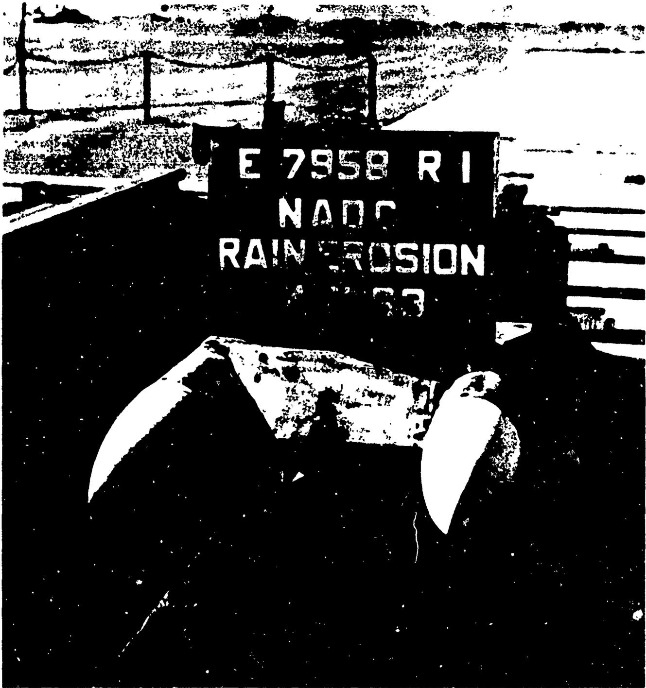
Figure 18. Pointed, Tip-glazed and Steel Tipped SCFS Domes Before Run #8.
