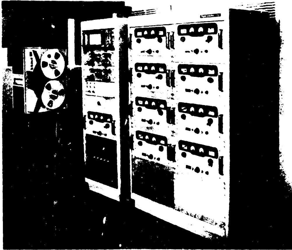
GROUND RECEIVING STATION
