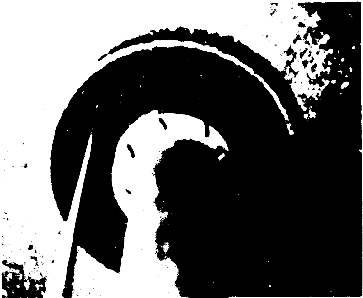
Fig. 33. Dome of pump riser in IS storage tank. Note severe corrosion in dome area. Other areas have been scraped.
