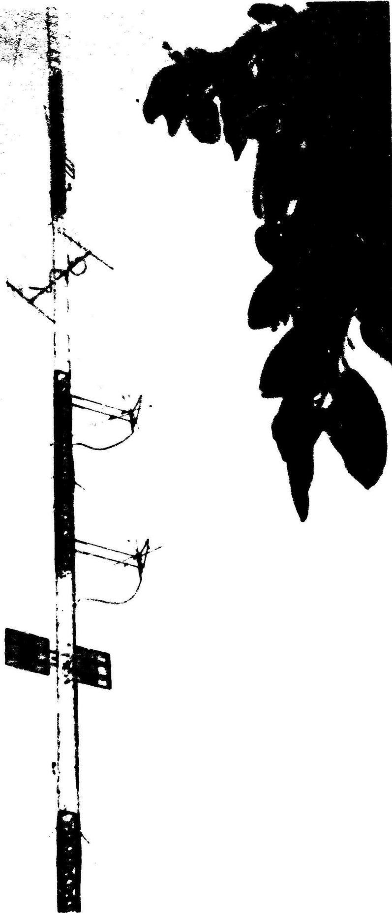
Figure K-18 View of Tower showing from Bottom Upwards; AN/TRC-24 Antennas, Two 50 MC Reference Receiving Antennas, Two UHF Data Link Antennas, and a 900 MC Receiving Test Antenna
