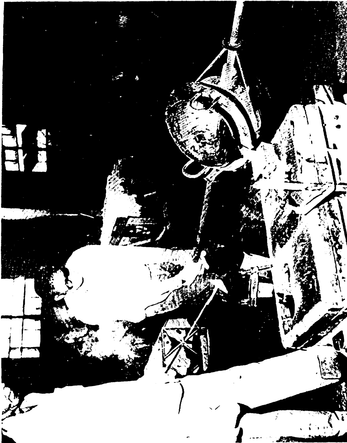
FIGURE 10 POURING ZQ64 MAGNESIUM ALLOY
