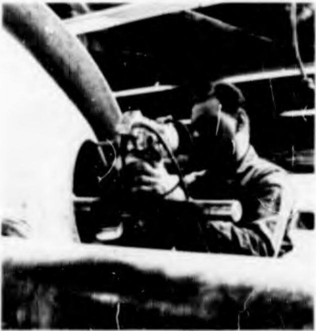
Figure 22. TU-226A Case Fabrication
