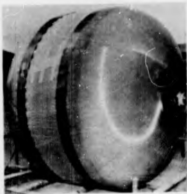
Figure 53. TU-228 Aft Dome Fabrication
