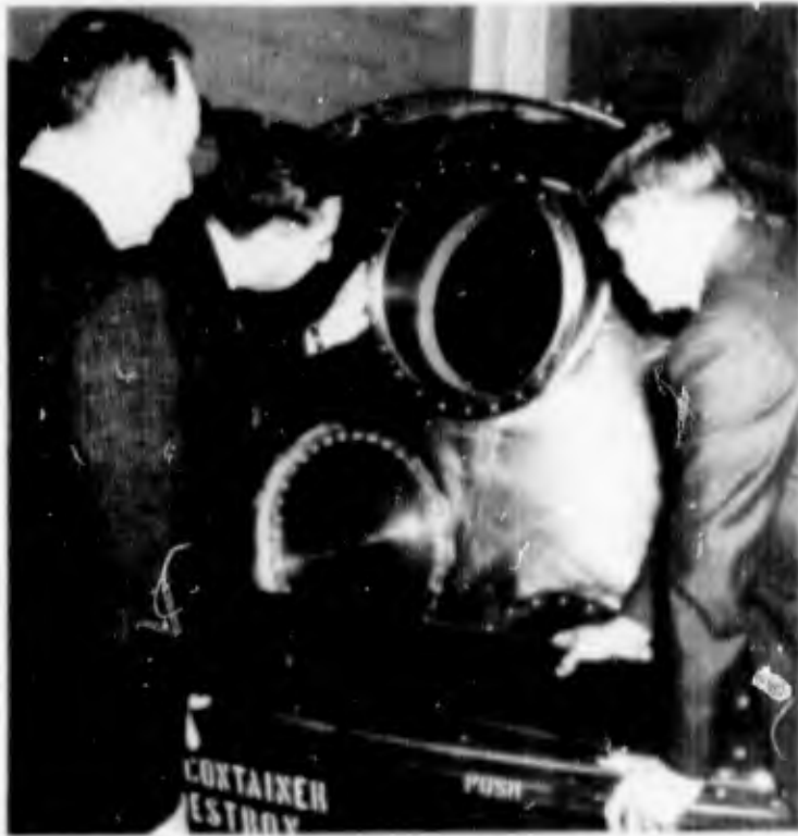
Figure 25. Completed TU-226B Case
