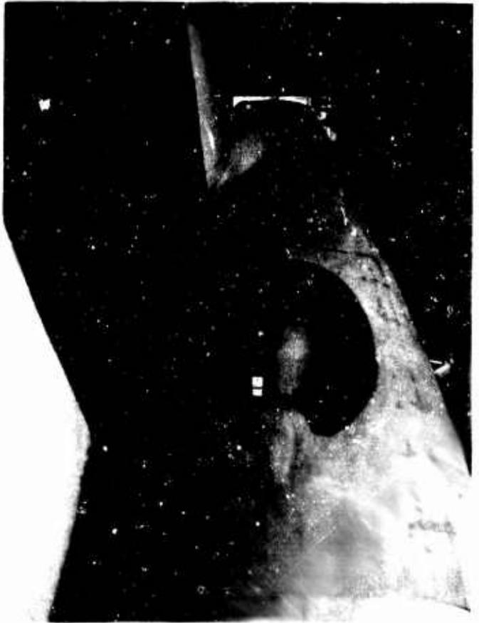
Fig. 2.01(b). PB4Y-2, A.T. No. 14, showing Erco port waist-turret with camera on gun.
