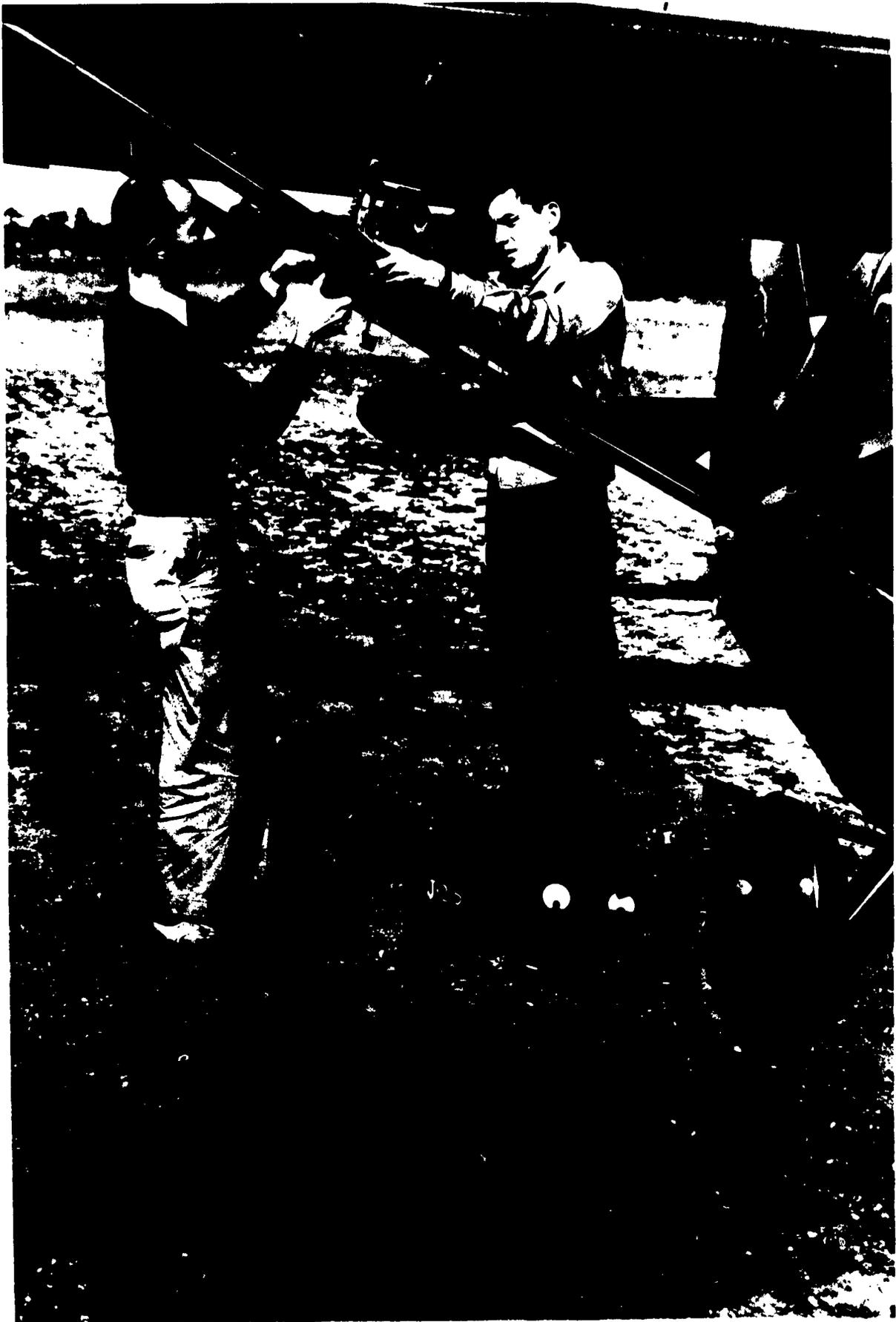
FIG. 1- PSYCHROGRAPH HOUSING BEING MOUNTED ON WING STRUT.
