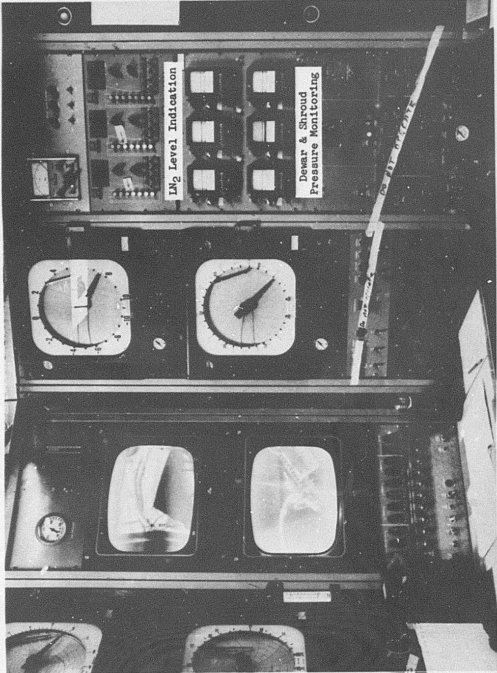
Figure 2-18 Radiation Effects Console in Reactor Control Room - Right Side
