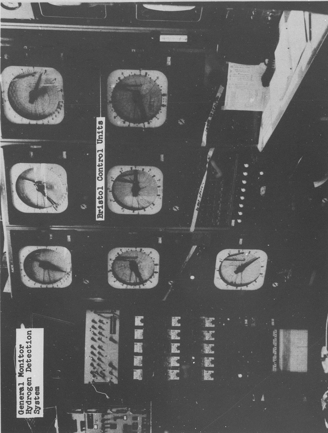
Figure 2-12 Radiation Effects Console in Reactor Control Room: Left Side
