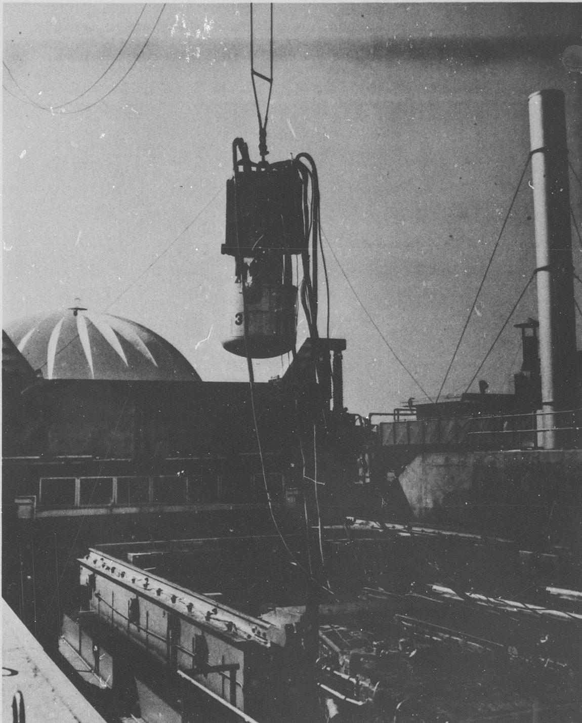
**Figure 2-6** Installation of AGC Cryogenic Materials Test Assembly
