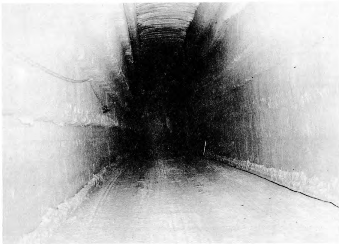
Figure 2. Snow tunnel (cut-and-cover type).
