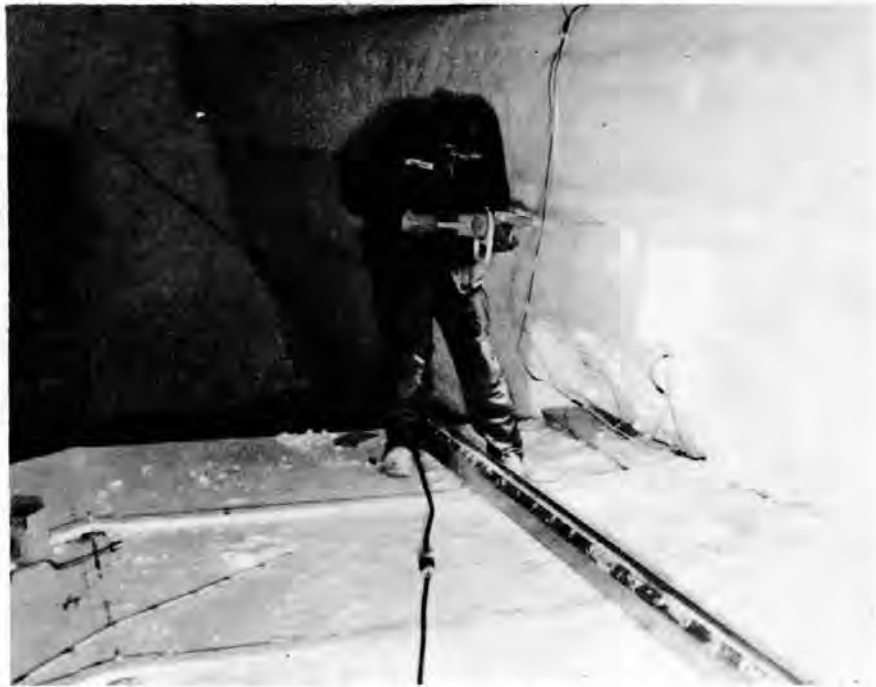
Figure 33. View from top of one of the T-5 buildings in a standard trench, showing a soldier using an electric chain saw to trim snow away from the building eave.
