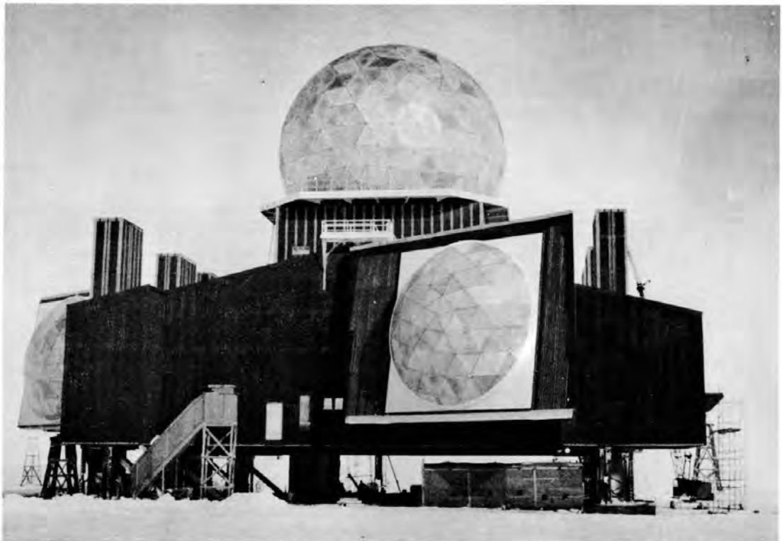
Figure 5. Texas Tower concept used in Greenland Ice Cap DEWline sites. Built-in jacking device permits periodic raising of structure as new snow accumulates.
