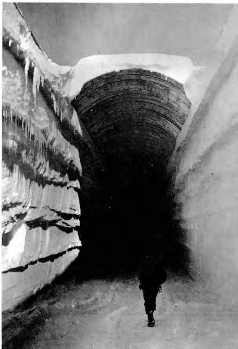
Figure 11. Undercut trench.
