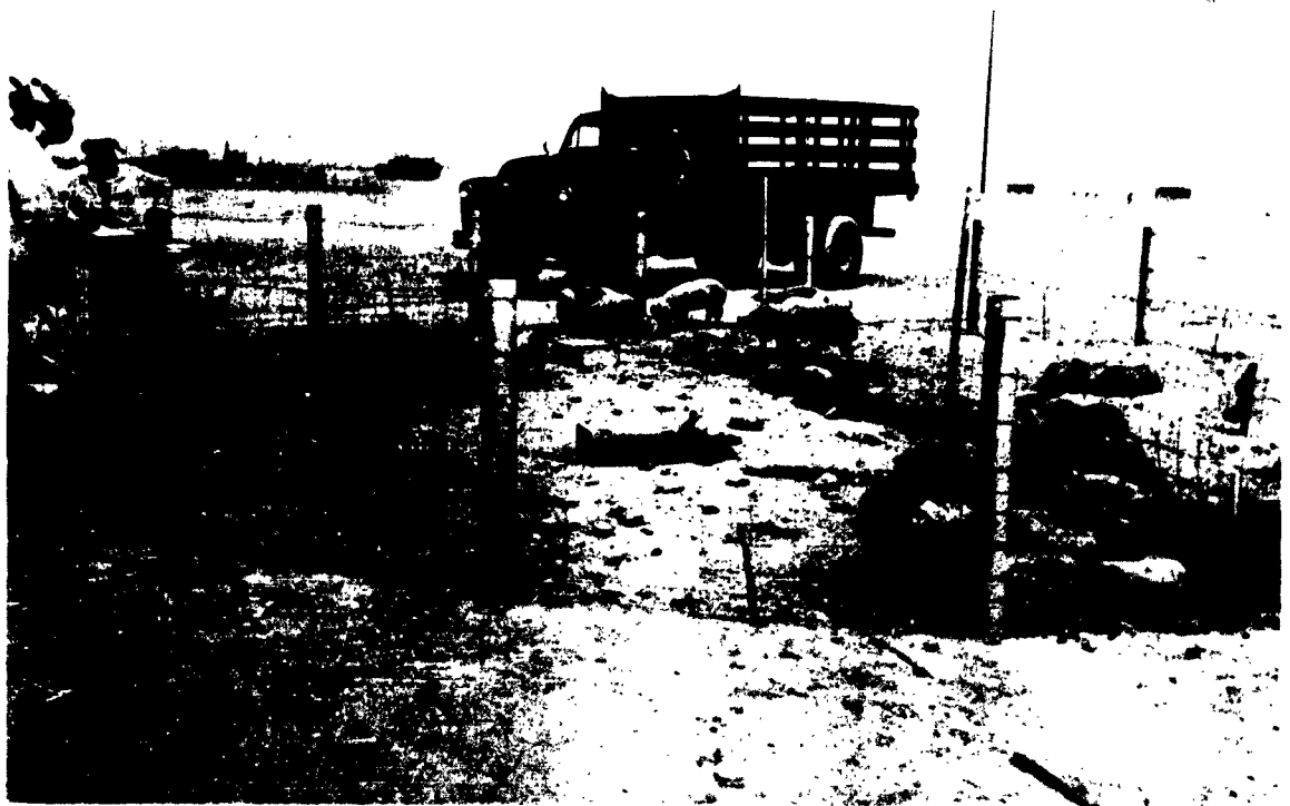
Figure 7.4 Postshot view of Station 5, showing little displacement of battlefield debris.
