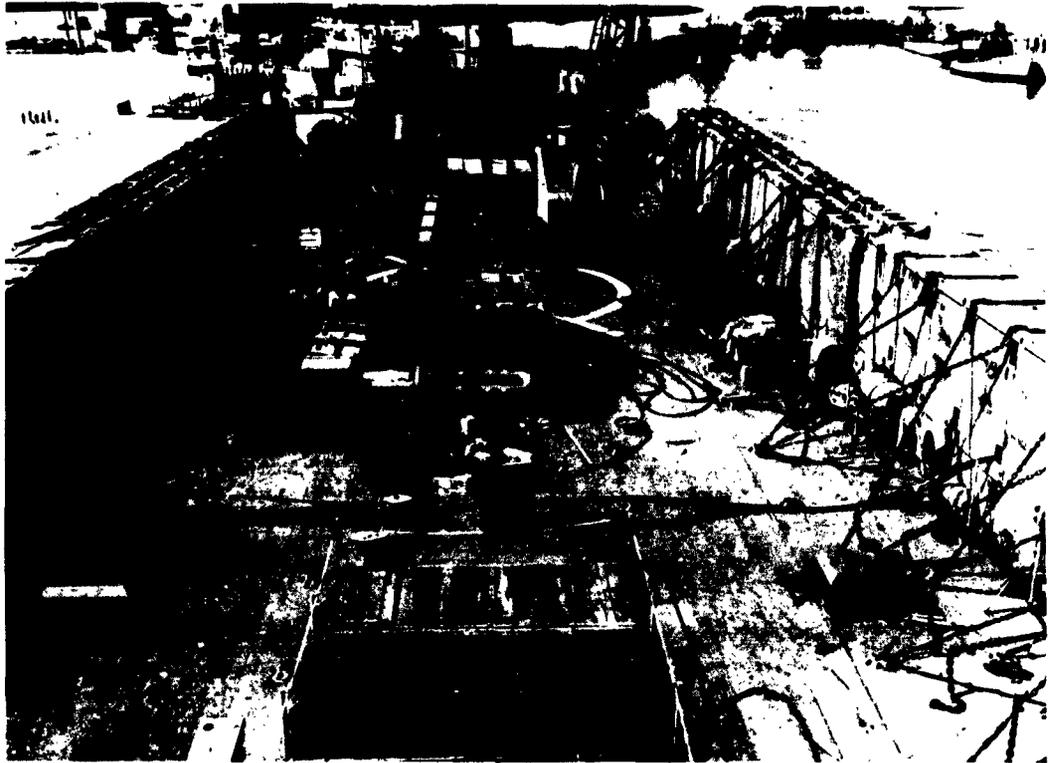
Figure 13. Four inflatable sections lashed for LST side-carrying.
