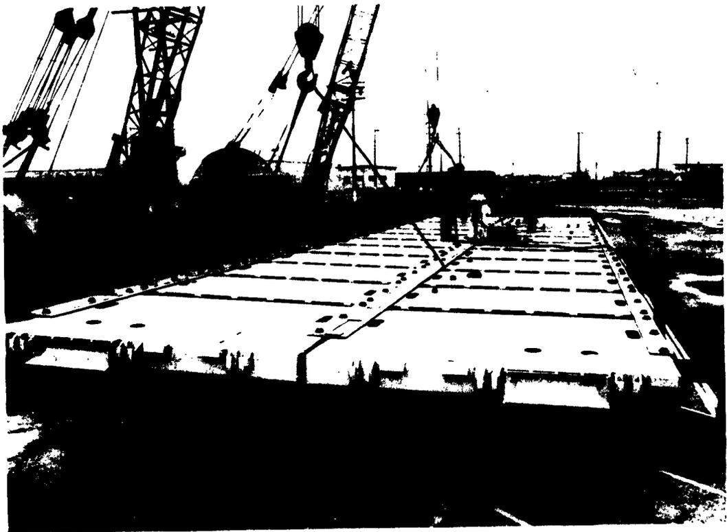
Figure 11. Strings being combined into complete sections.
