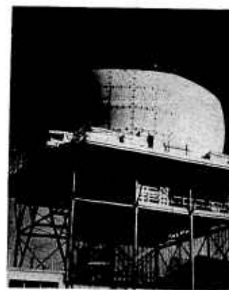
Radome, Distant Early Warning Radar Installations (Mobay)
