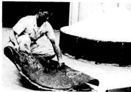
Fig. 13. Folding of heat shield
