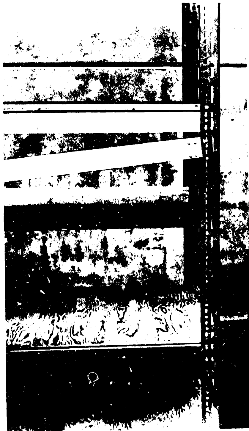
Fig. 6 Slotted Angle Unit Showing Attachment of Side Rails
