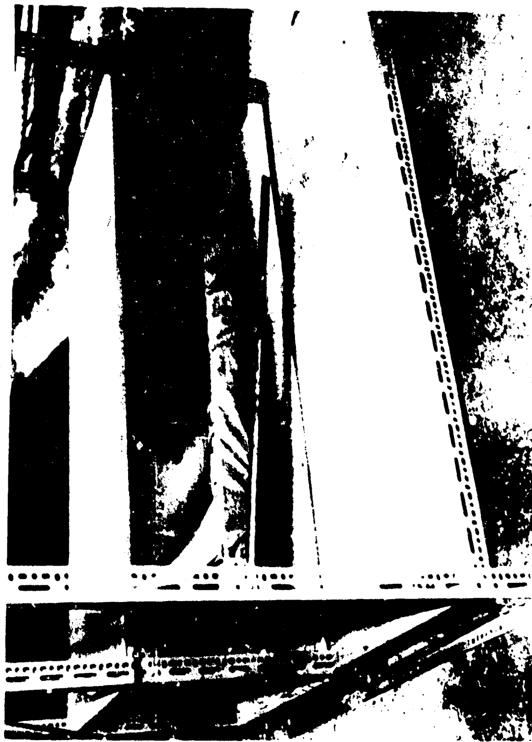
Fig. 3 Slotted Angle Unit Showing Bolted Construction and Hairpin Clip for Fabric
