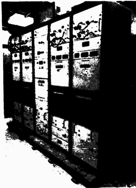
Figure 6, New Automated Receiving systems
