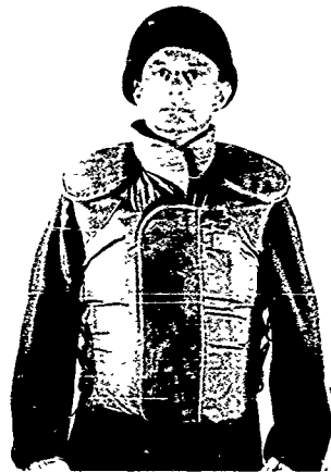
Figure 13. T62-5 Composite Titanium/Nylon Armor Vest
