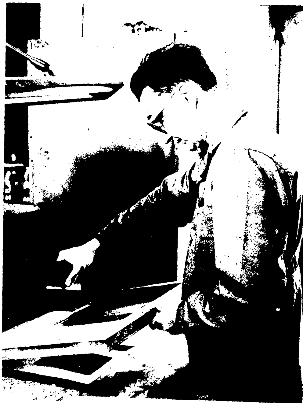
Figure 1. Applying Circuit Pattern by Silk Screen Method.
