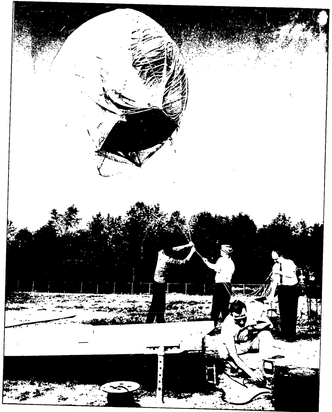
Figure 2. Ground Plane Installation
