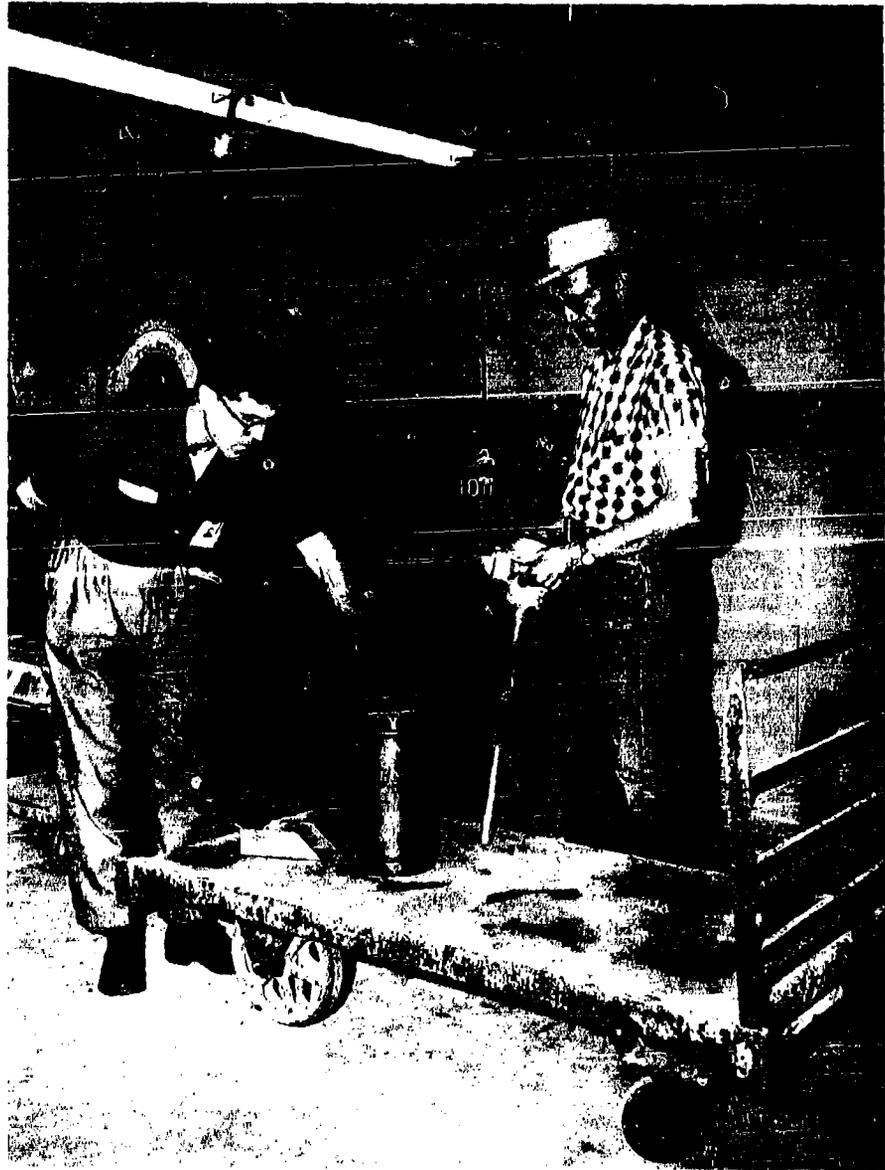
Figure 4. Placing steel grid in cylindrical mold.
