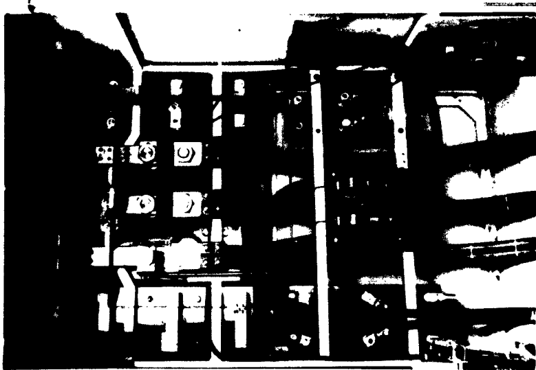
Figure 6. 2-Mw Power Supply Disconnect Cubicle (Rear View)
