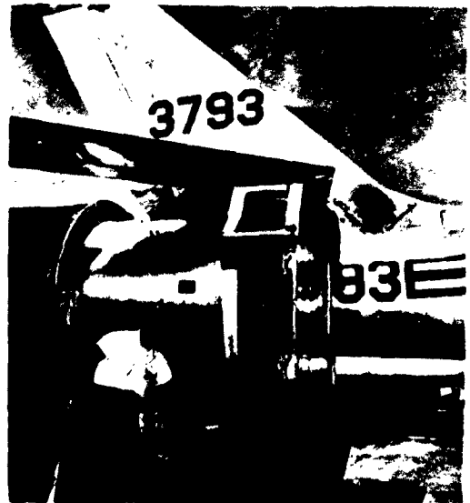
(c) COUPLING AND SECONDARY AIR INTAKE - PRODUCTION MODEL
