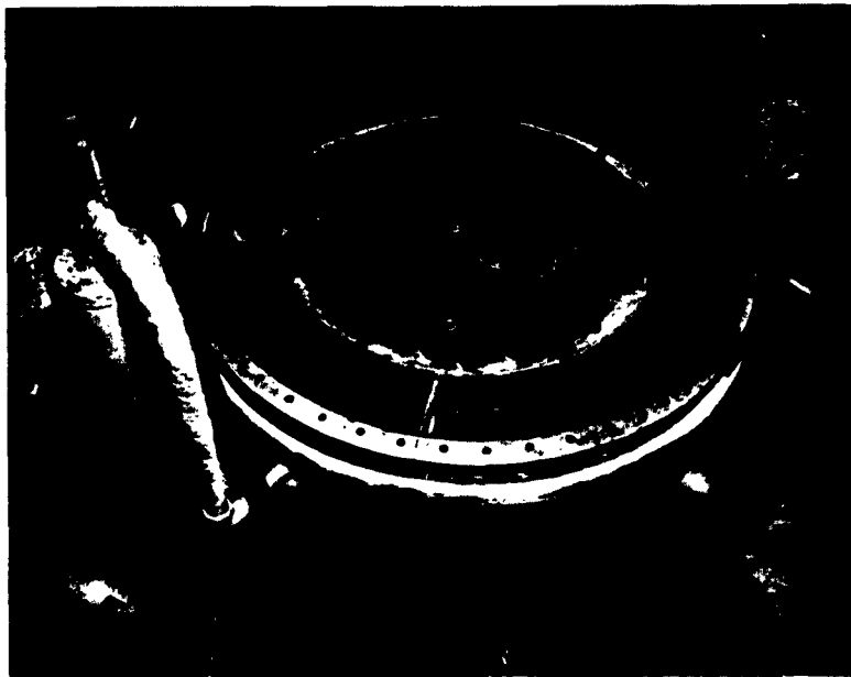
Figure 2. Top tube sheet showing compressor discharge end on bottom, right.
